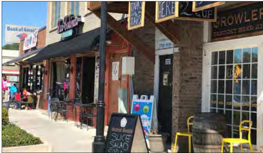
This older section of downtown Tucker today provides an excellent example of zero lot line development.
