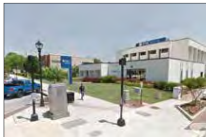
PNC Bank was built set back from Main Street.
