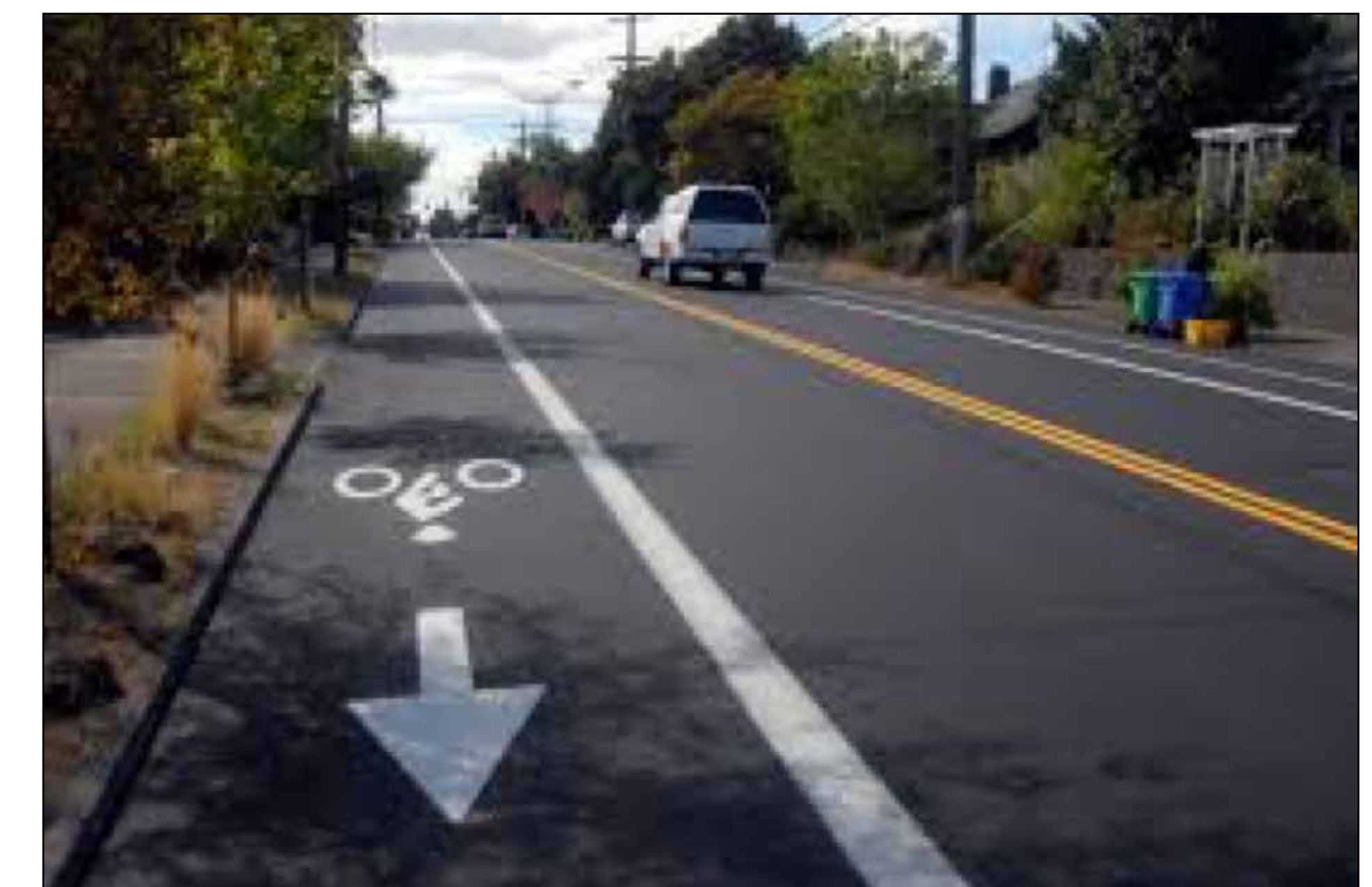
Typical on road bike lane and sidewalks
