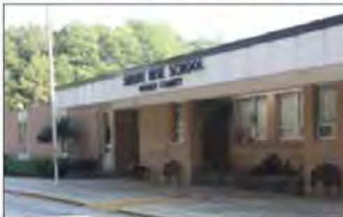
Northside of Hugh Howell potential site for new Smoke Rise Elementary
