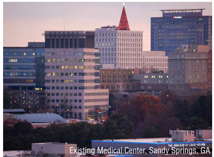
Existing Northside Hospital, Sandy Springs, GA
