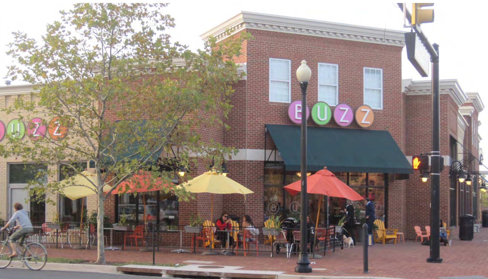
Single-story commercial building with faux second story to reinforce the pedestrian scale (Alexandria, VA)
