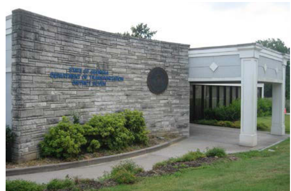
GDOT District 7 Office
