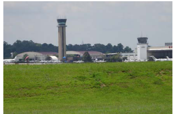
Airport Control Tower
