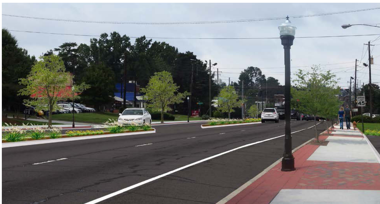
After: Peachtree Boulevard with Aesthetic Improvements
