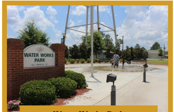
Water Works Park
