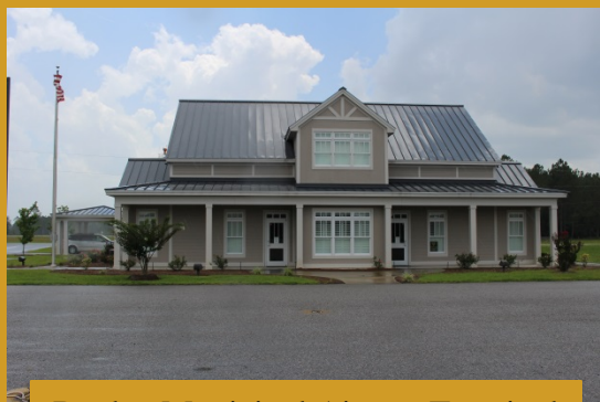
Baxley Municipal Airport Terminal
