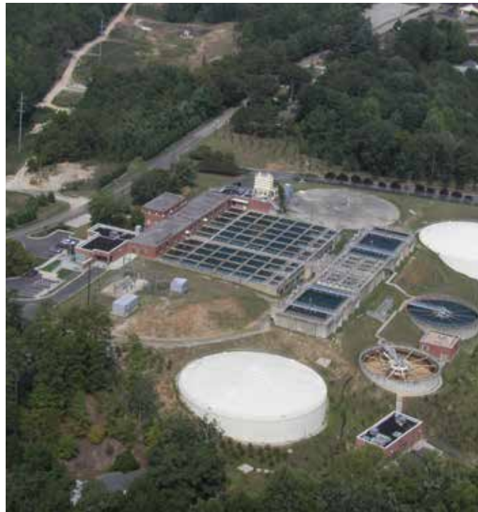
Riverside Water Treatment Plant
