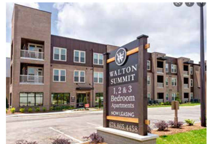
Example of a multi-family building
