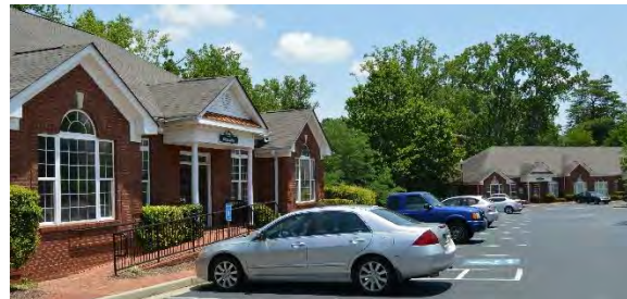
Existing office space in the city
