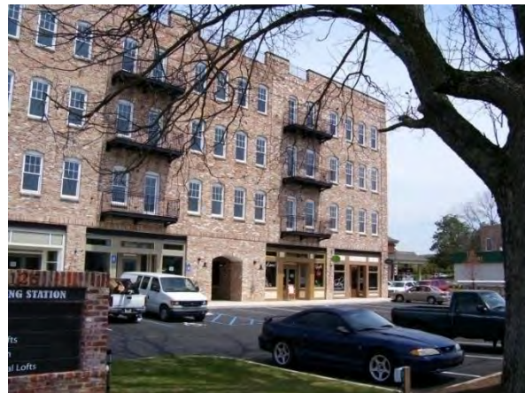
Cumming Station is in the CBD and provides lofts for downtown living
