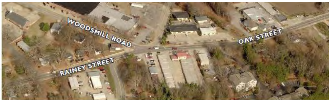
Aerial view of Oak / Rainey Corridor
