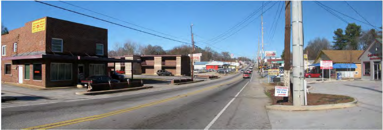
Atlanta Highway Corridor near Ray Street looking north - Before
