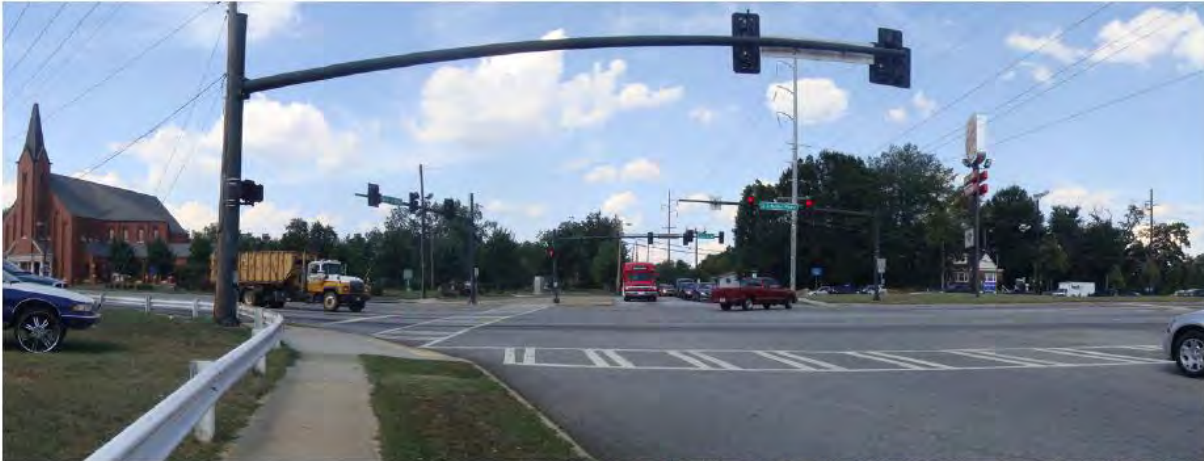
Before - Martin Luther King Jr. Boulevard and E E Butler Parkway Intersection looking northeast
