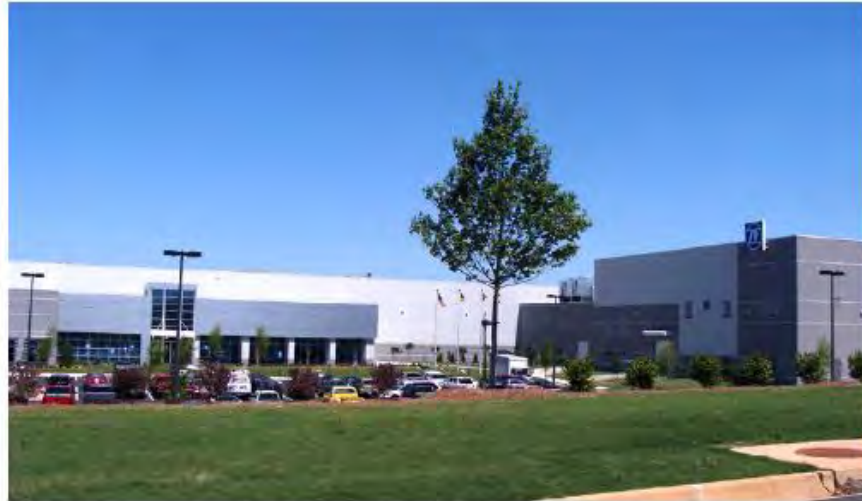
Existing Industrial Development
