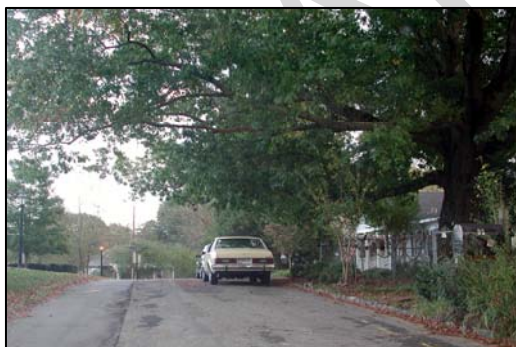
The historic street design of the Mill Village reflects the utilitarian function of the area as a home to mill workers. Streets were narrow, many without curbs, some with irregular granite stone curbing and no sidewalks.
