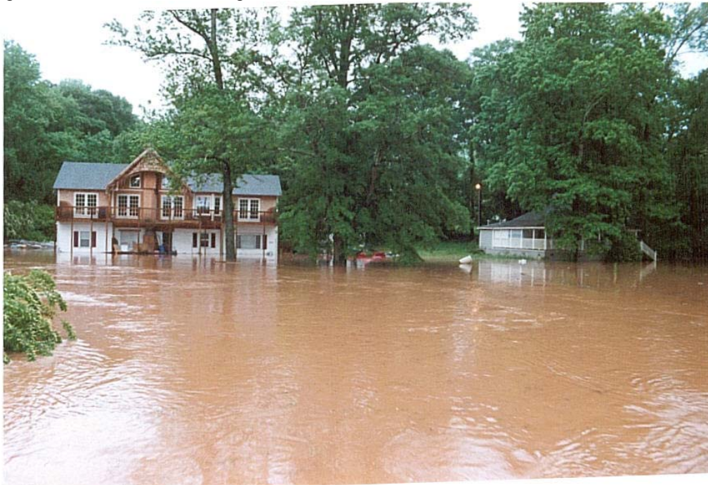
Figure 100: Picture – Flooding in Flood Plain
