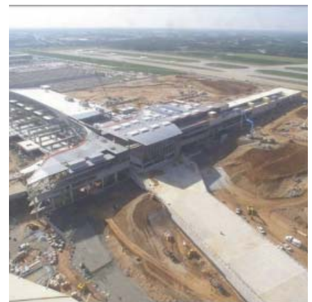
The Maynard H. Jackson International Terminal under construction.
