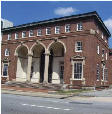
The Crum and Foster buildings is one the historic buildings in Midtown.
