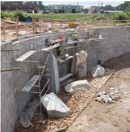
Historic Old Fourth Ward Park under construction, NPU M.
