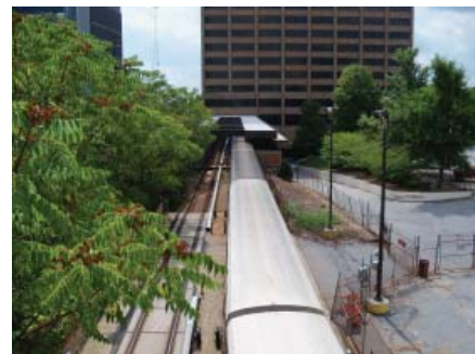
Georgia State MARTA station from the Courtland Street Bridge.
