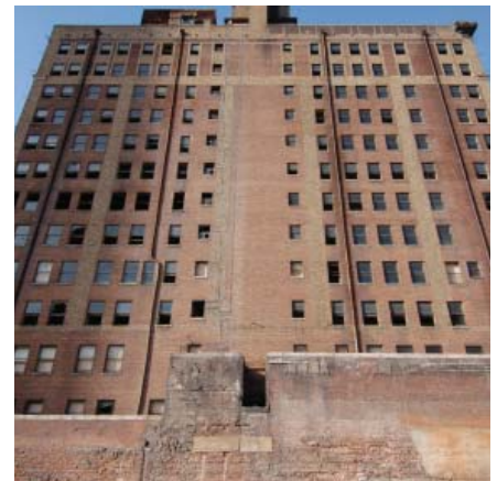
The Medical Arts Buildings is an endangered historic building.
