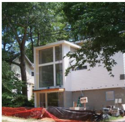
New Single family home construction in Candler Park, NPU N.
