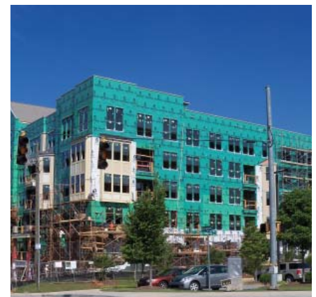
Multi-Family building under construction.
