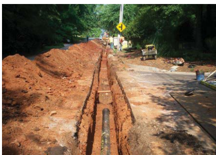
Water line replacement on North Highland.
