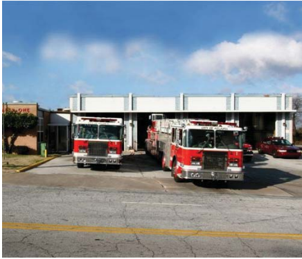
Fire Station 1 on Elliot Street, NPU M.
