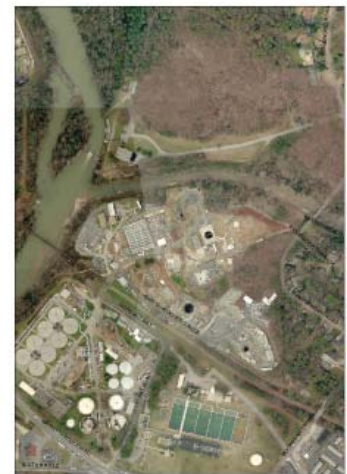
Chattahoochee Water Treatment Plant.
