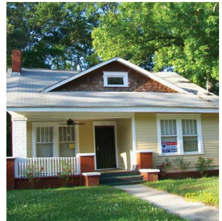
This house on Elbert Avenue in the Adair Park Historic District was purchased with NSP funds and was part of the 106 Review process, NPU V.
