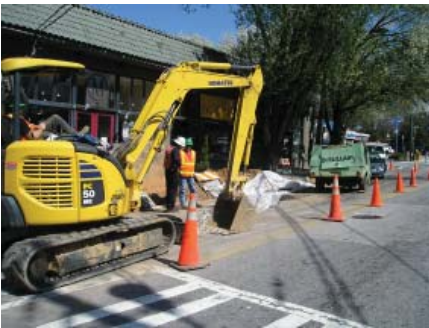
Water main replacement, part of the Clean Water Atlanta infrastructure upgrades
