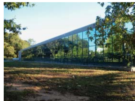
Clear Creek CSO Overflow Facility near Piedmont Park.
