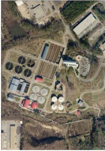
Utoy Creek Water Reclamation Center.
