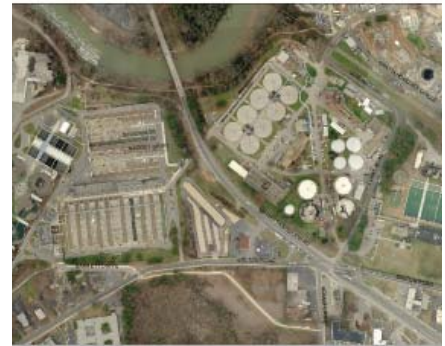
RM Clayton Water Reclamation Center
