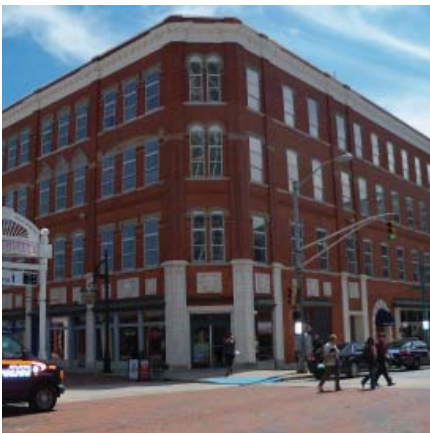
The Atlanta Development Authority office is located downtown.
