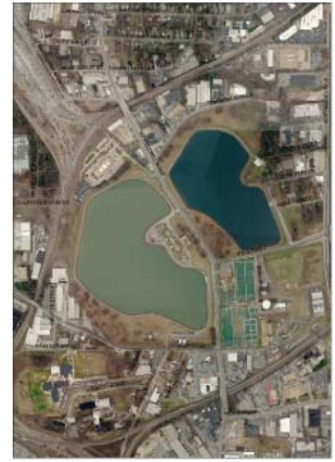
Hemphill WTP Reservoirs.
