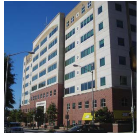
The Atlanta Public School headquarters.
