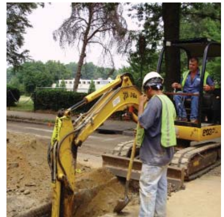
Water main replacement on Charles Allen Drive, NPU E.
