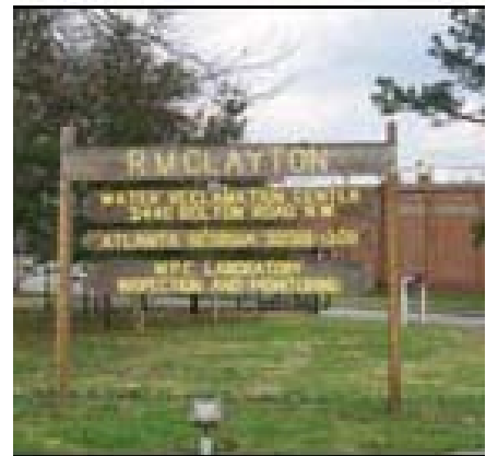
Entrance to the R.M. Clayton Water Reclamation Center.
