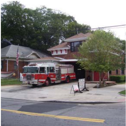
Station 19 on North Highland Ave. NPU F.
