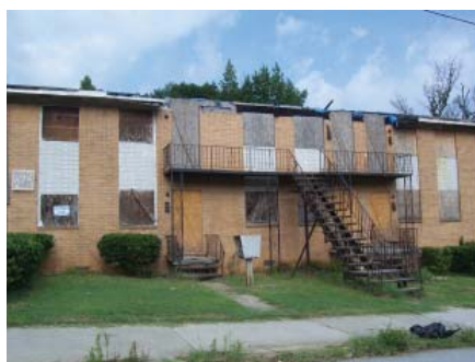
Multi-family residential in deteriorated condition, NPU L.
