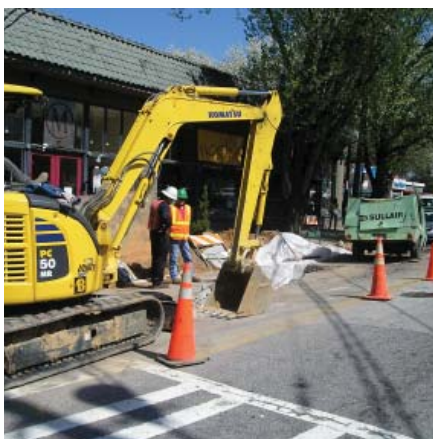
Water line replacement on North Highland and Virginia Avenue.
