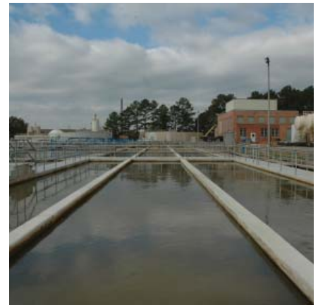
Chattahoochee Water Treatment Plant.
