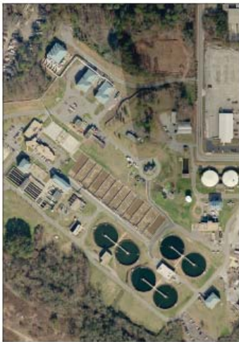
South River Water Reclamation Center.
