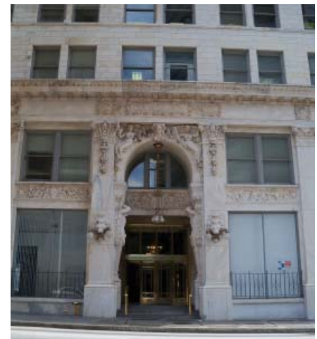
Candler Building detail, a Landmark designated building in downtown, NPU M
