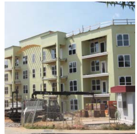
Rental housing units under construction.
