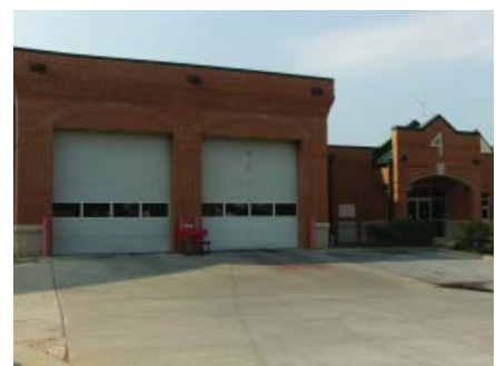
Fire Station 4 on Edgewood Avenue, NPU M.
