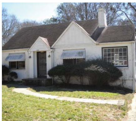
This house on Allegheny Street was purchased with NSP funds, NPU T.
