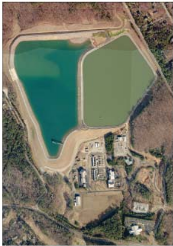
Atlanta Fulton County Water Treatment Plant in the City of Johns Creek.
