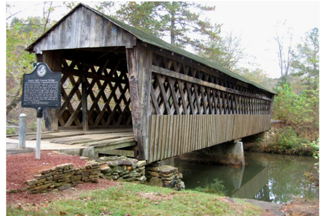
Figure 5: Poole's Mill Bridge after Restoration
