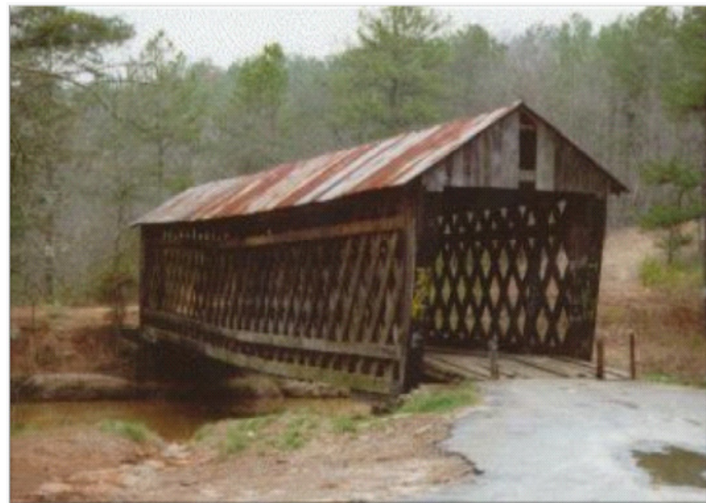
Figure 4: Poole's Mill Bridge prior to Restoration
