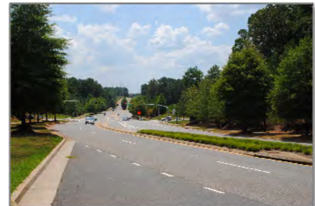
Transportation improvements are a key strategy to improve the quality of life and economic competitiveness for the North Fulton CID.
