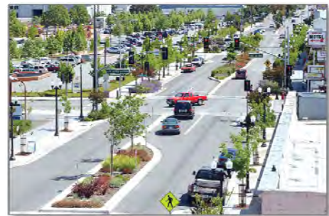
Transportation enhancements along the South Main Street Corridor could support new development while making it more walkable by adding wider sidewalks, more pronounced cross walks, on-street parking, street trees, a tree-lined and landscaped median and buildings built to the edge of the sidewalk, as shown in this example photo.
