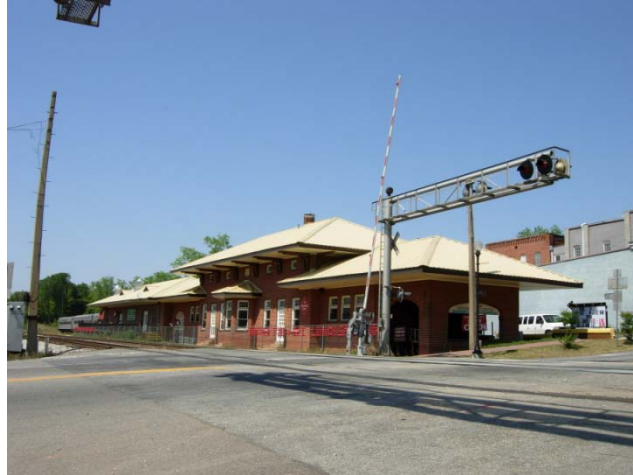
Historic Train Depot, now commercially owned. Part of the Downtown Business District, 5-21-07
