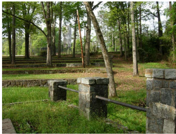
WPA-Era Outdoor Amphitheater 1916 concrete water tower in background, 4-4-07
