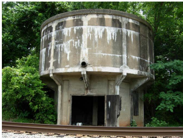
Historic RR Water Tank, owned by CSX, 5-28-10
