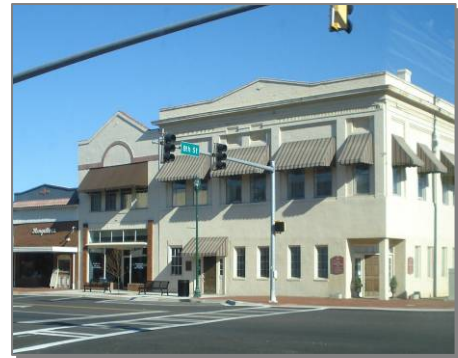
Two-story, corner historic buildings in Downtown character area
