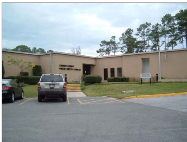
The Camden County Public Safety complex is located on the courthouse square in Woodbine.
