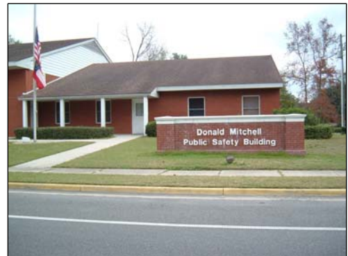
Camden County leases the Donald Mitchell Public Safety building from the City of Woodbine.
