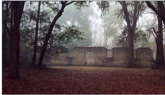
John Houstoun McIntosh Sugarworks, located on Spur 40, is notable for being the first animal-powered horizontal sugarmill in Georgia. (Photo courtesy of Tara Fields)
