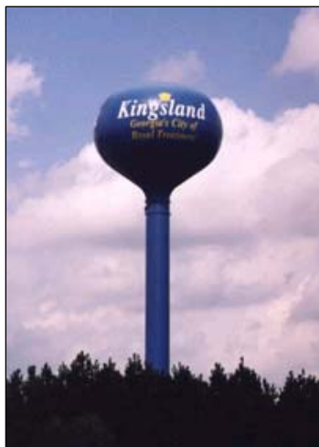
The City of Kingsland has very distinctive water storage facilities.
