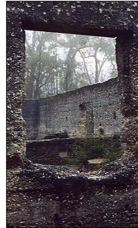
The Sugarworks ruins are an example of poured tabby walls based upon the “Spalding method” and the use of whole oyster shells in manufacturing a coastal concrete. (Photo courtesy of Tara Fields)
