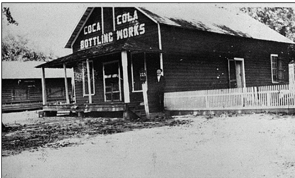
Coca-Cola Bottling Works building in 1914. (Photo courtesy of Vanishing Georgia, Georgia Division of Archives and History, Office of Secretary of State)
