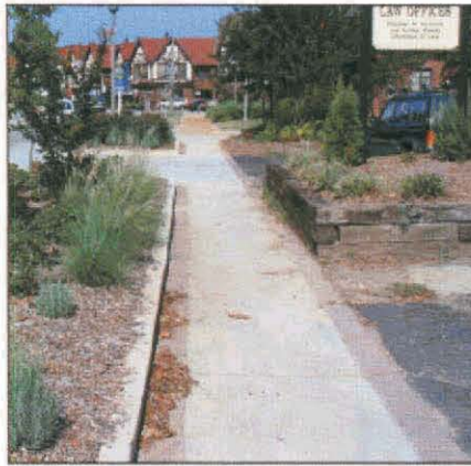
Sidewalk near City Hall constructed as part of streetscape program.
