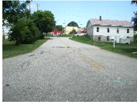
Main St. (NW toward Atlanta Highway)
