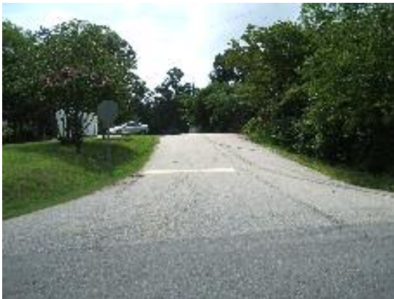
Oak Street (E from Holland Dam)
