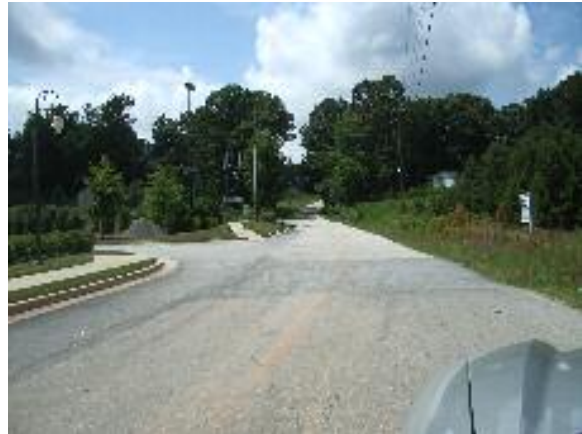
Holland Dam Rd (S) from Spout Springs Rd.
