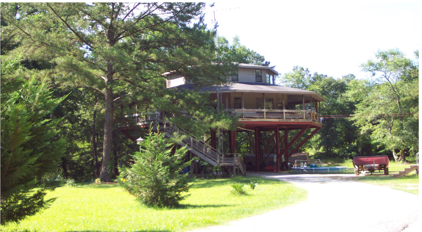
A more elaborate version of raising the house to evade flood water
