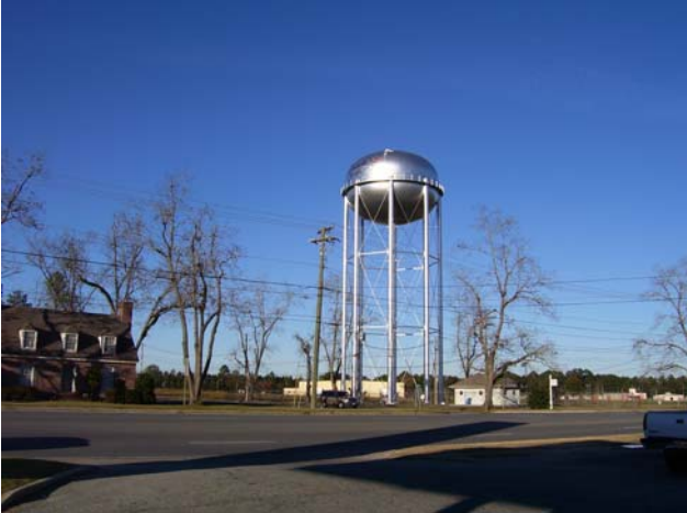
Water Tank, Pavo Road, Thomasville
