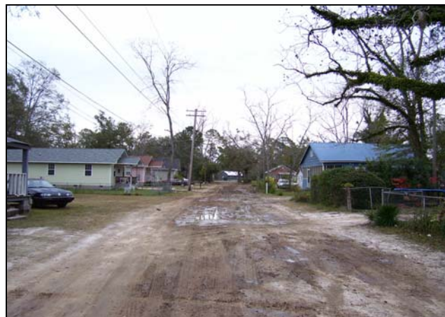
One of several unpaved or substandard roads within Thomasville’s neighborhoods
