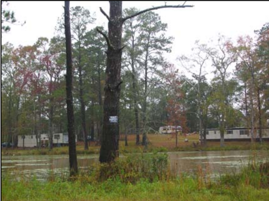
Dilapidated trailers near Powell Drive and Inman Roads
