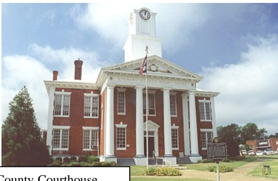
Stewart County Courthouse
