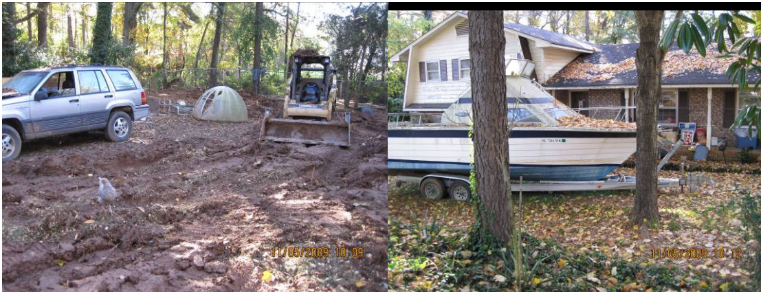
A property in the Urban Redevelopment Area with code and maintenance issues.
