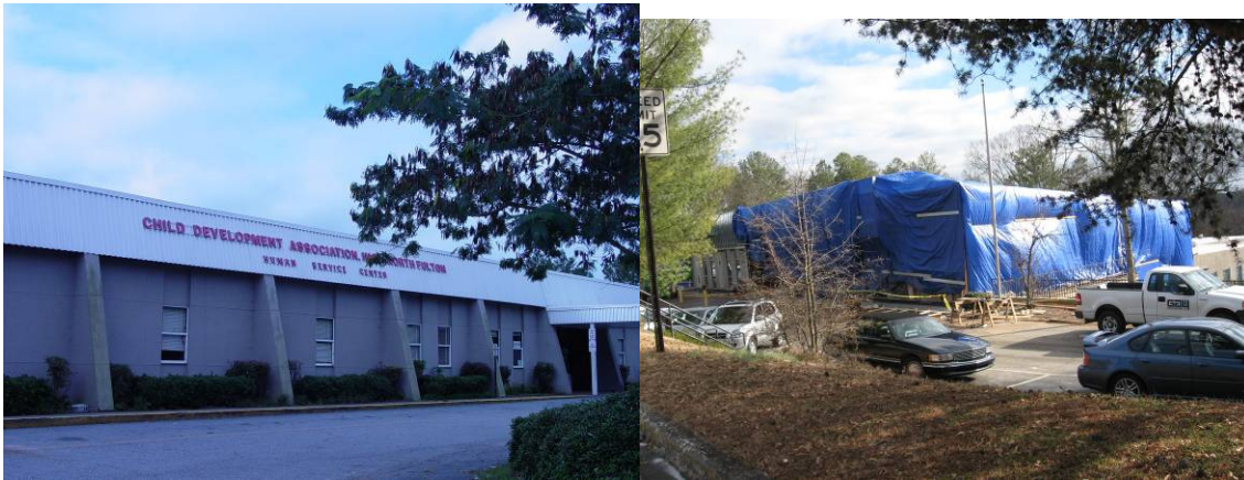
North Fulton Human Services Center is under renovation.
