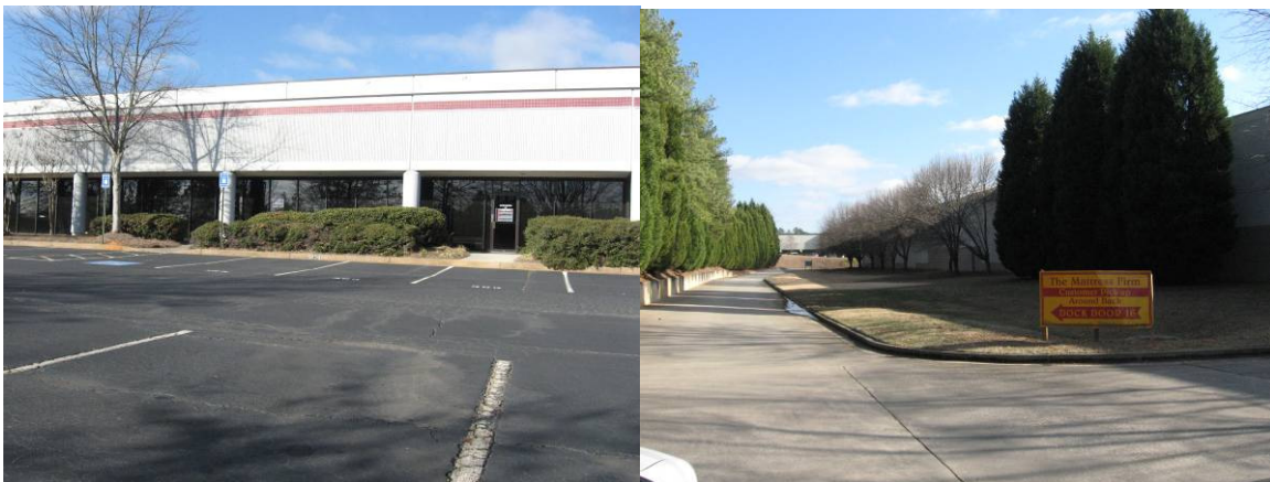
Northfield Business Center
