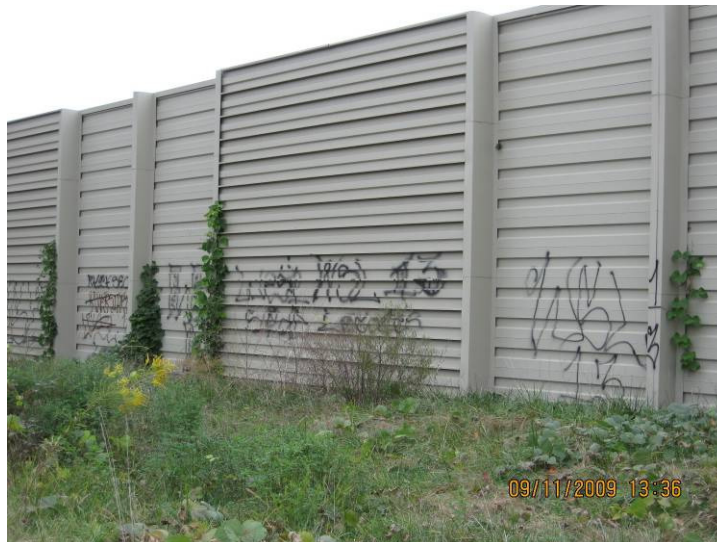
Old Holcomb Bridge Road graffiti
