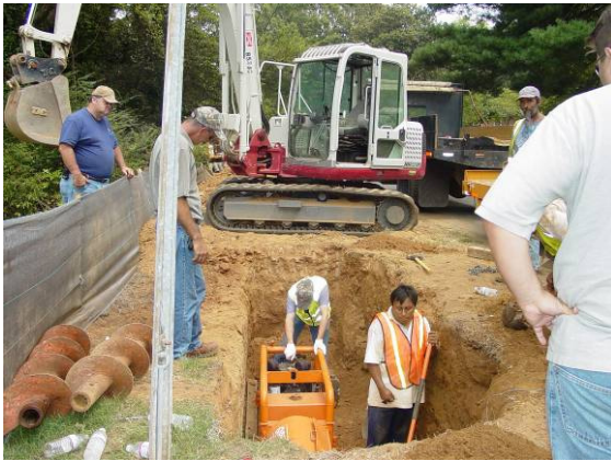
CDBG funded Waterline installation in URA
