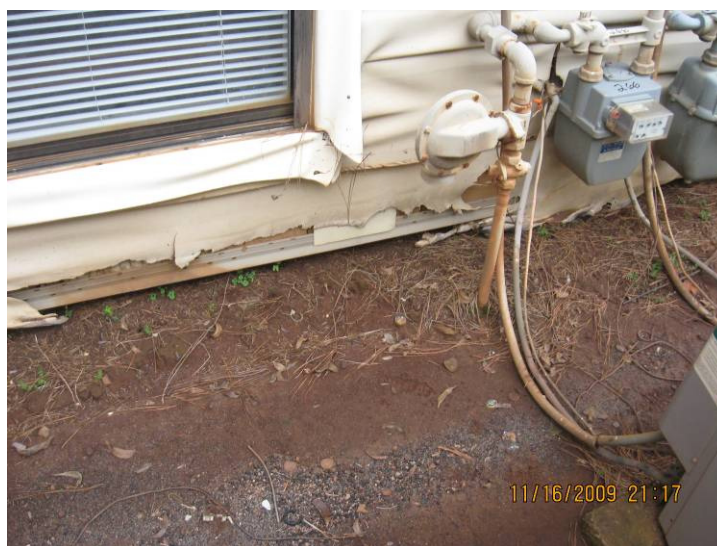
Damaged siding
