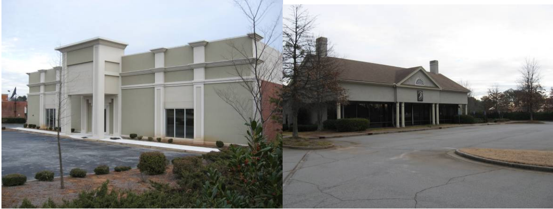
Former Drexel Heritage store, vacant over 5 years
