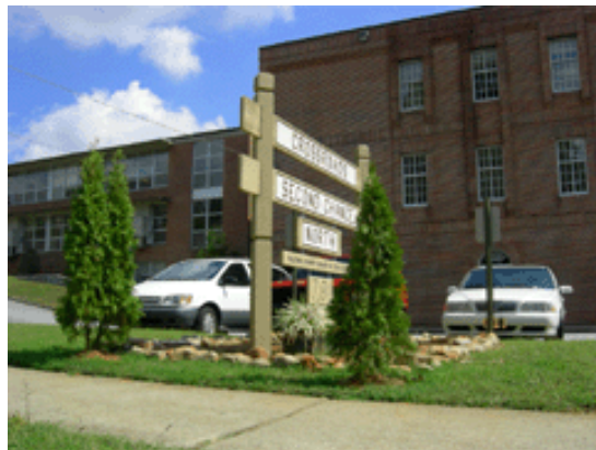
Crossroads Second Chance School on Mimosa Blvd
