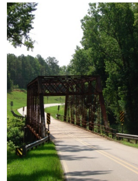
Figure 9 Salem Road Bridge
