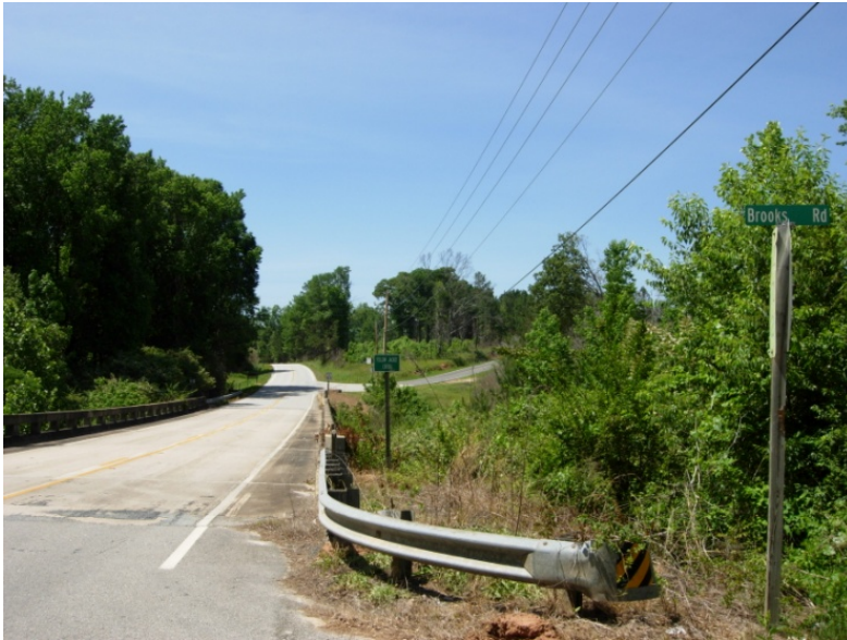
Westside Creek Bridge, May 19, 2010
