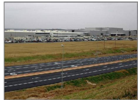
Kia Automotive Manufacturing Plant under construction in West Point
