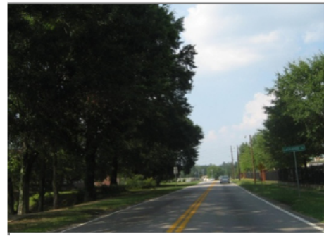
The cross-section for US-29 north from SR-18 does not include sidewalks or bike lanes
