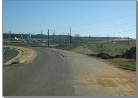
Kia Boulevard adjacent to the Kia plant, shown under construction in 2007
