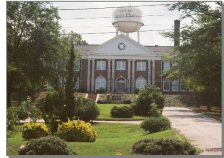
Historic school in West Point
