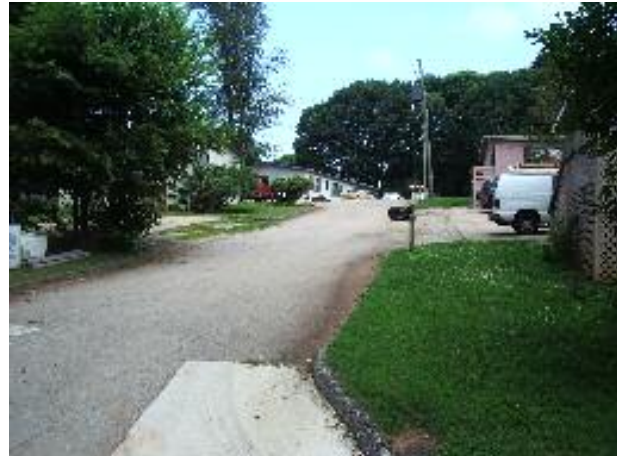
Concrete Patch of Asphalt Road Lorimar Court
