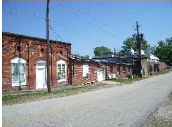
Redevelopment Potential along Railroad Avenue
