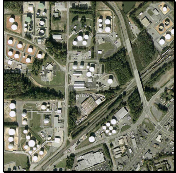
Doraville tank farm industries: Aerial Photo
