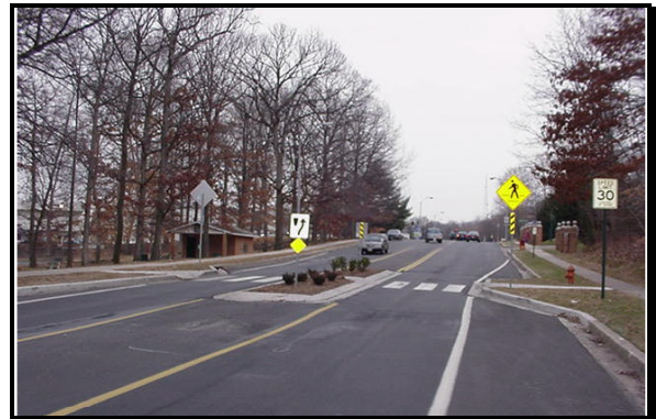
Bulb-outs and pedestrian island as traffic calming measures
