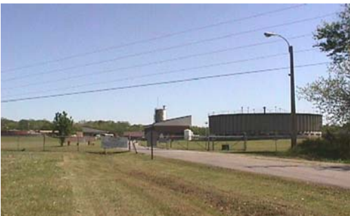
Poplar Street Treatment Plant
