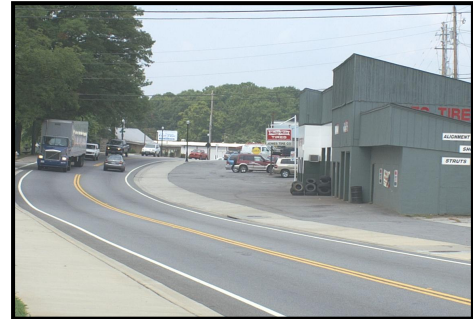
Figure 2-11: South Main Street Commercial Corridor.
