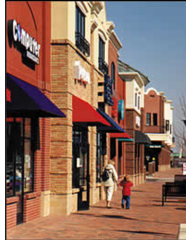
Detailed architecture on strip commercial facades
