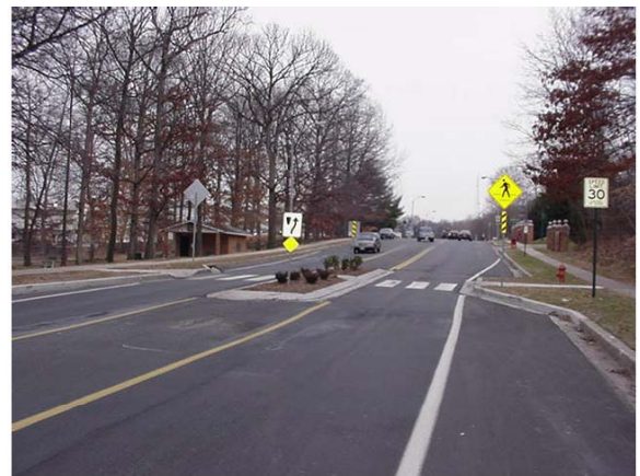
Bulb-outs and pedestrian island as traffic calming measures
