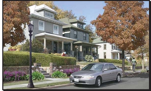
Traditional Neighborhood Development: Small setbacks, sidewalks, and on-street parking
