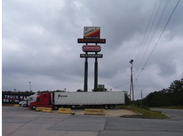
Current development in the I-75 corridor at SR 36 consists of highway-oriented development such as this truck stop.
