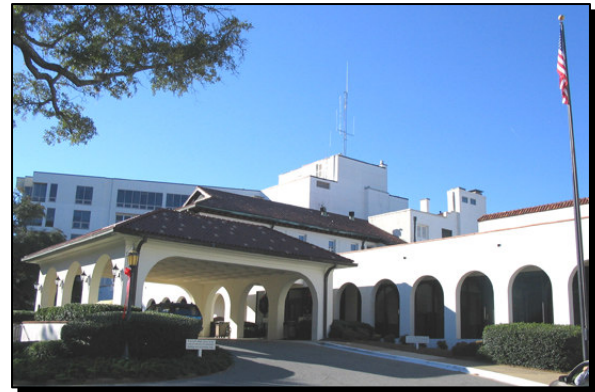
Archbold Hospital Complex
