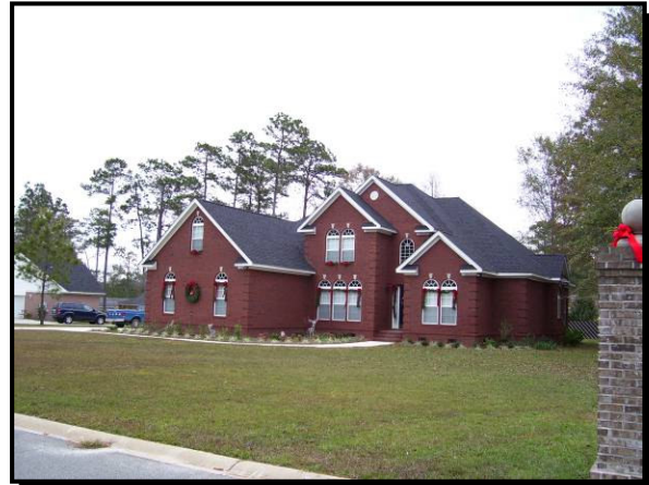
Housing Construction in Thomas County
