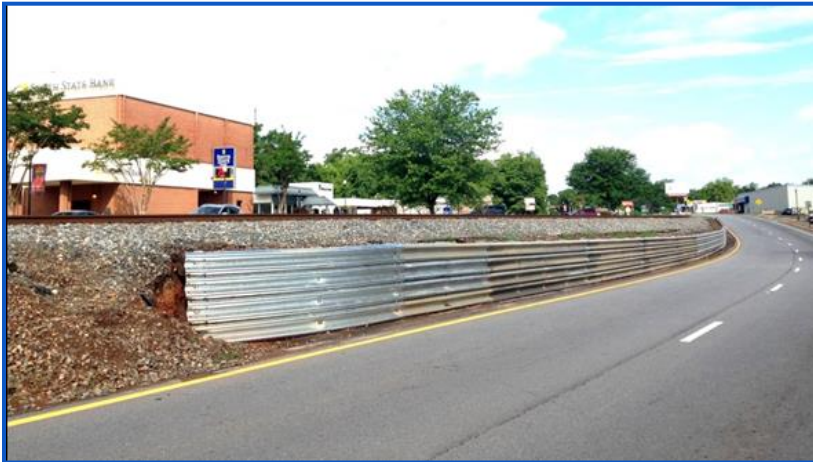
Retaining wall repair on Broad St.
