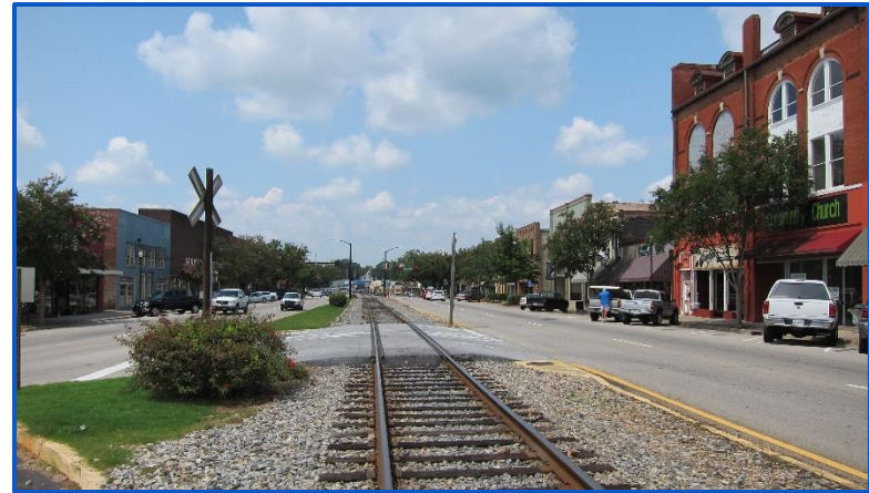
Historic buildings and the railroad tracks are defining characteristics of the downtown that are valued by residents.
