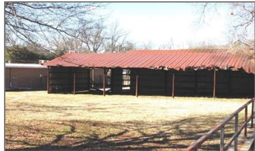
Pole barn structure in downtown Commerce.
