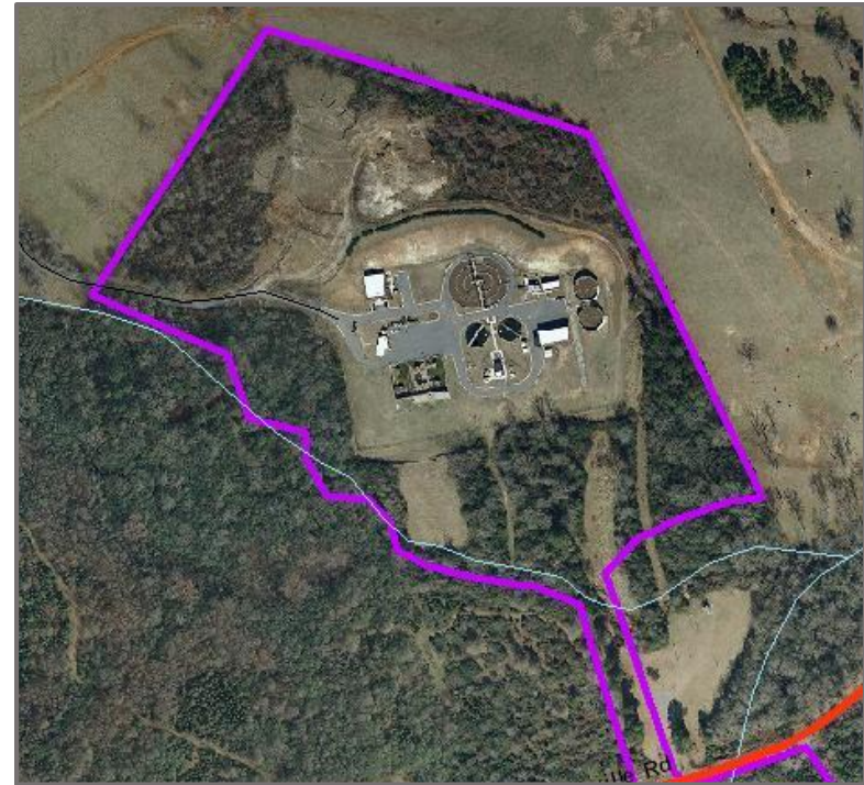
Commerce's treatment plant is an example of a special, single-use character area.
