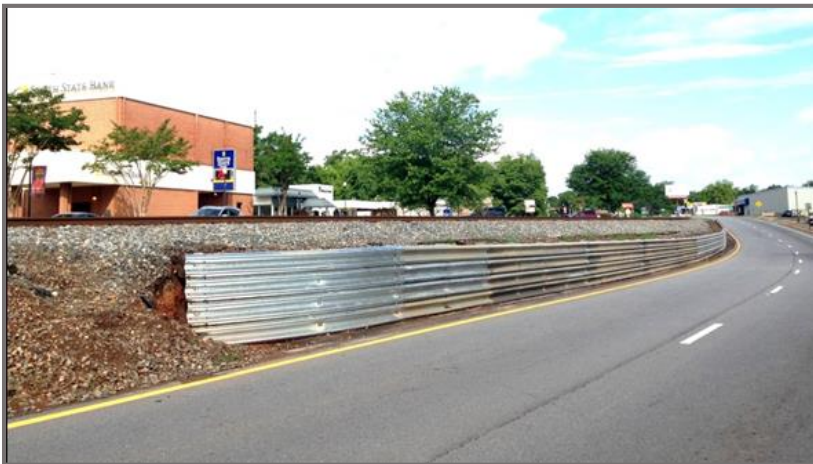
Retaining wall repair on Broad St.
