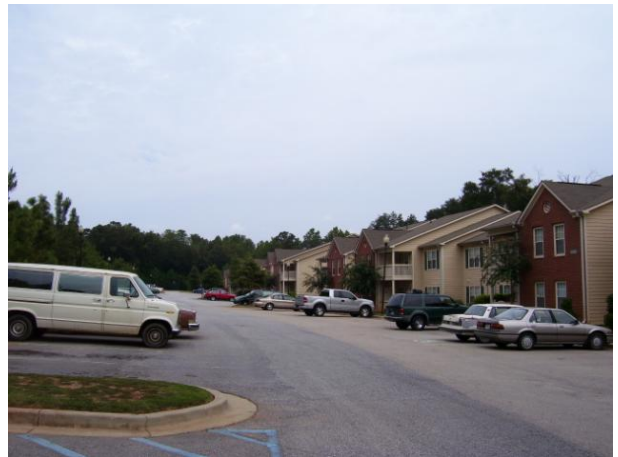
Apartment Complex in Commerce
