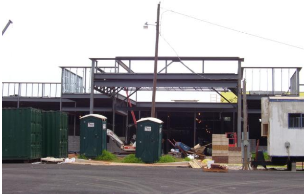
New School Under Construction, Main School Campus
