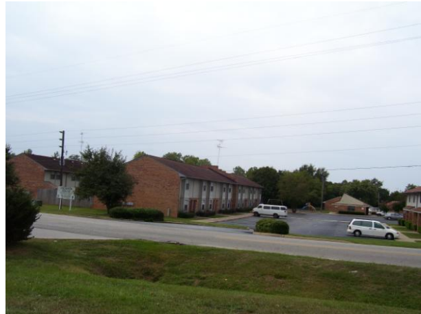
Jackson Hills Apartments, along B. Wilson Road, just outside the city limits of Commerce
