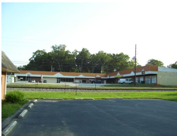
Older shopping centers such as this one along Maysville Road (SR 98) may be threatened by newer retail development opportunities
