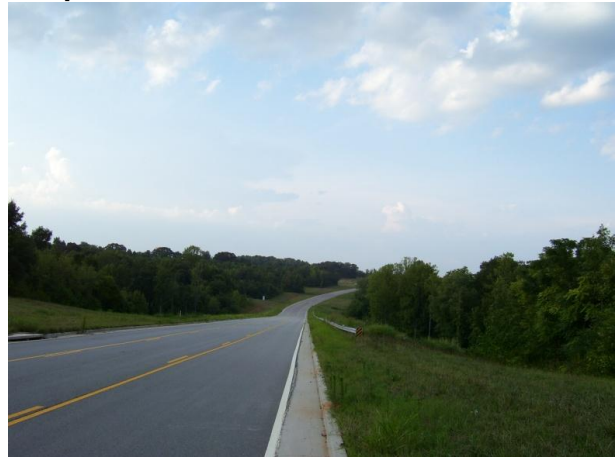
Steve Reynolds Industrial Boulevard (looking north) is ready for industrial development
