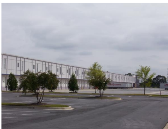
Huge potential exists for Commerce to attract warehousing and distribution centers, such as this one developed in the I-85 corridor west of Commerce, in unincorporated Jackson County.
