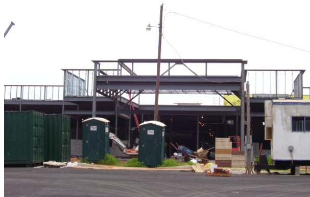
New City School Under Construction, 2009
