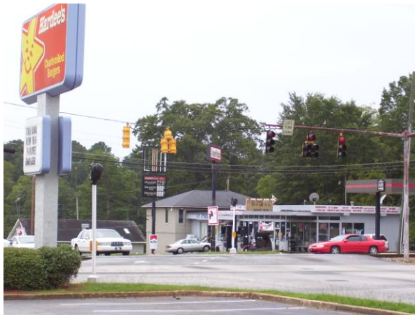
Sign blight: Portable sign on roof; ground sign with panel missing
