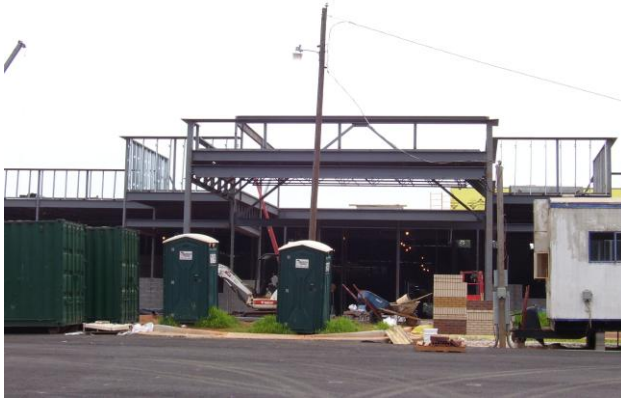
New School Under Construction, Main School Campus
