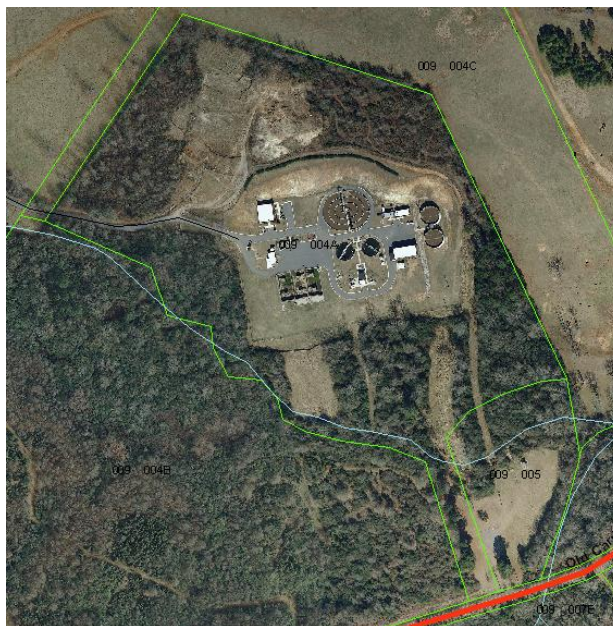
Sewage Treatment Plant, Aerial View
