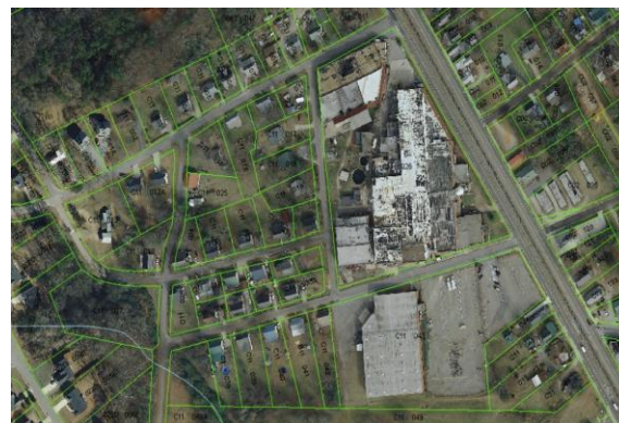
Mill Village, U.S. Highway 441 Bus. south of downtown core
