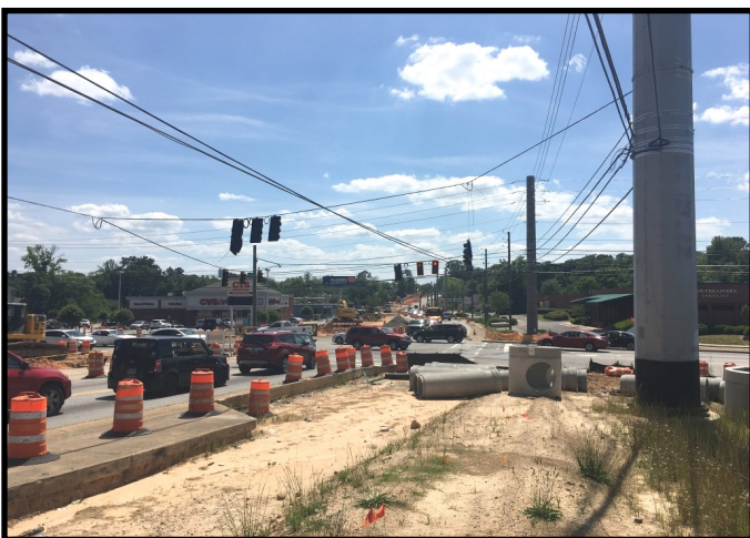
Talbotton Road Widening Project
