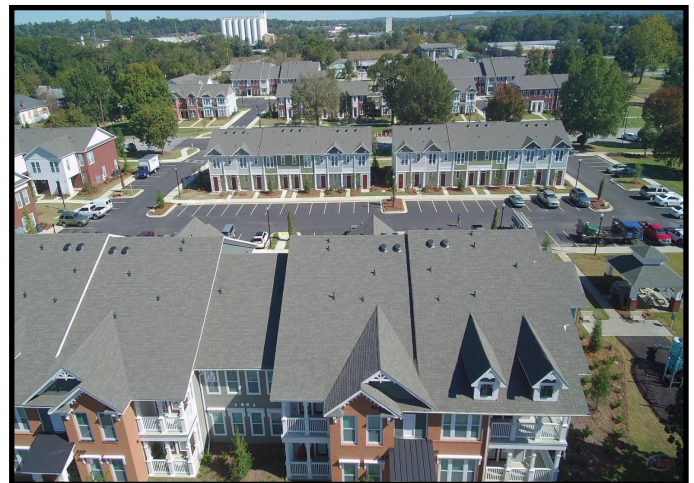
Aerial view of Arbor Point Apartments
