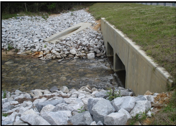
Lindsey Creek passing through a culvert
