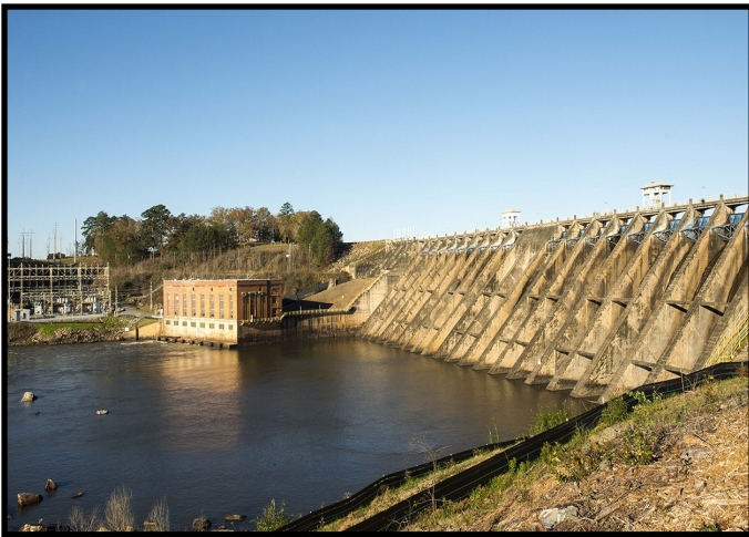
Bartletts Ferry Dam (north of Columbus, GA)
