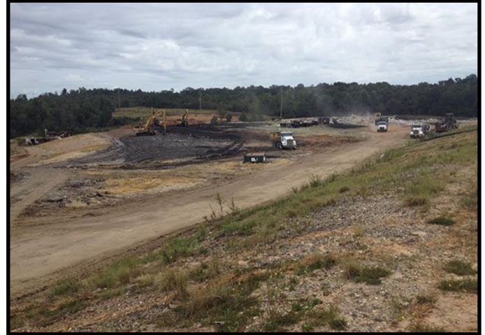
Pine Grove Landfill
