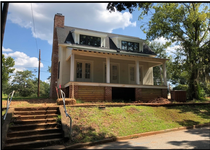
New single family housing under construction
