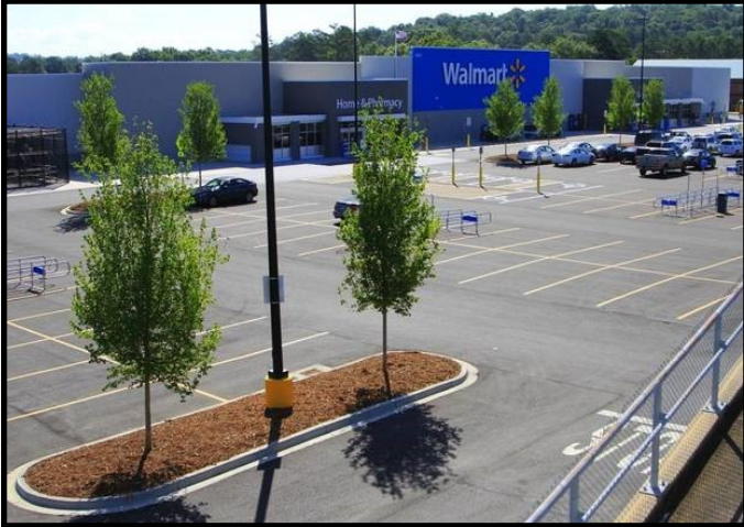
Walmart On Victory Drive
