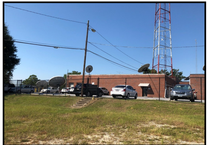
WRBL Station and Broadcast Tower
