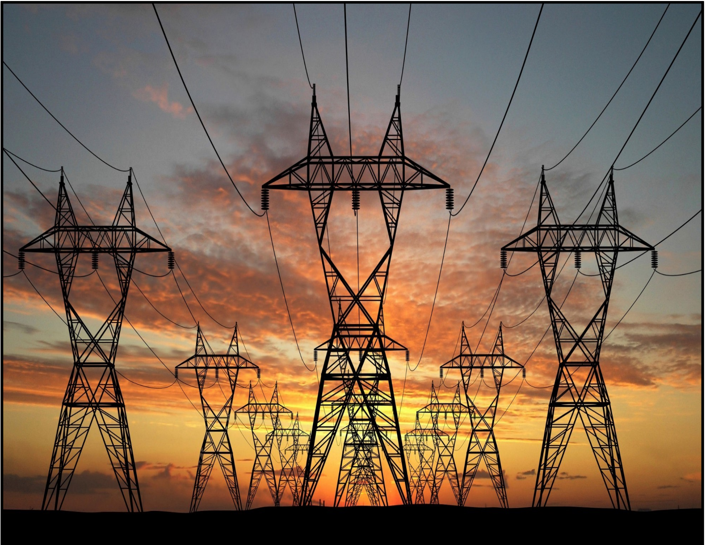
High Voltage Transmission Lines
