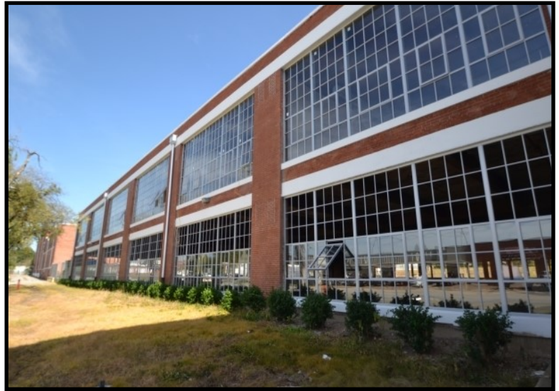
Swift Mill Apartments
