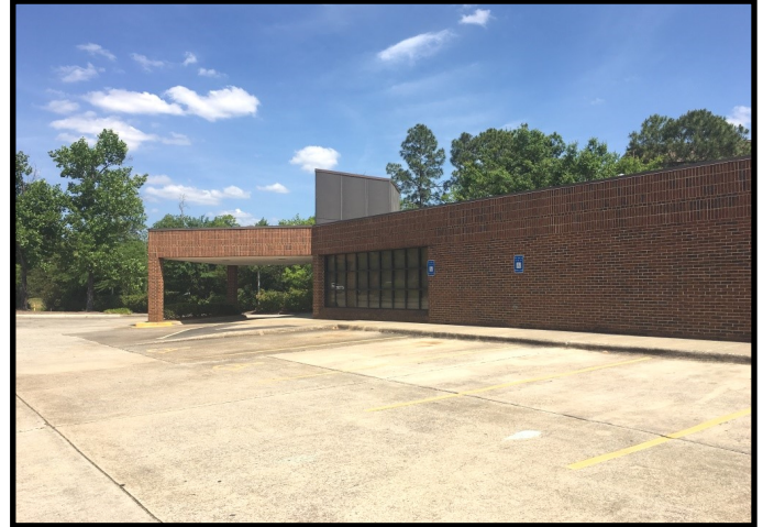
Vacant Medical Office Building
