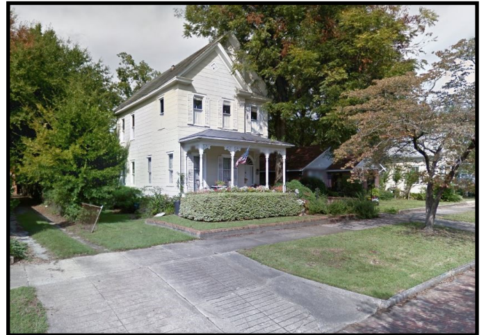
Single Family Residence in the Historic District
