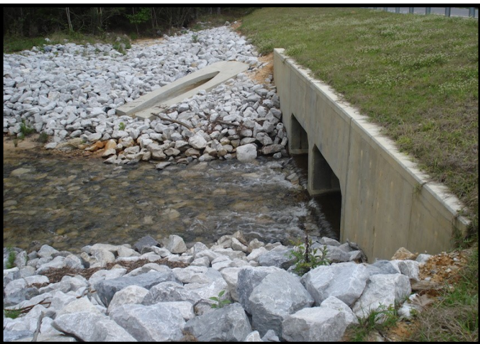
Lindsey Creek passing through a culvert
