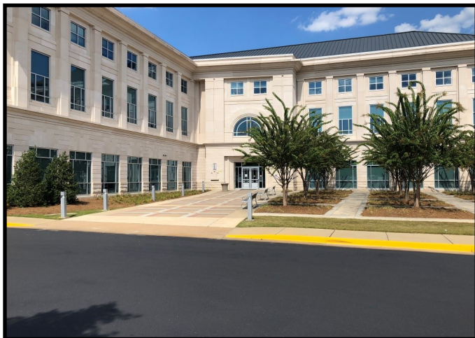
Muscogee County School District Admin. Building
