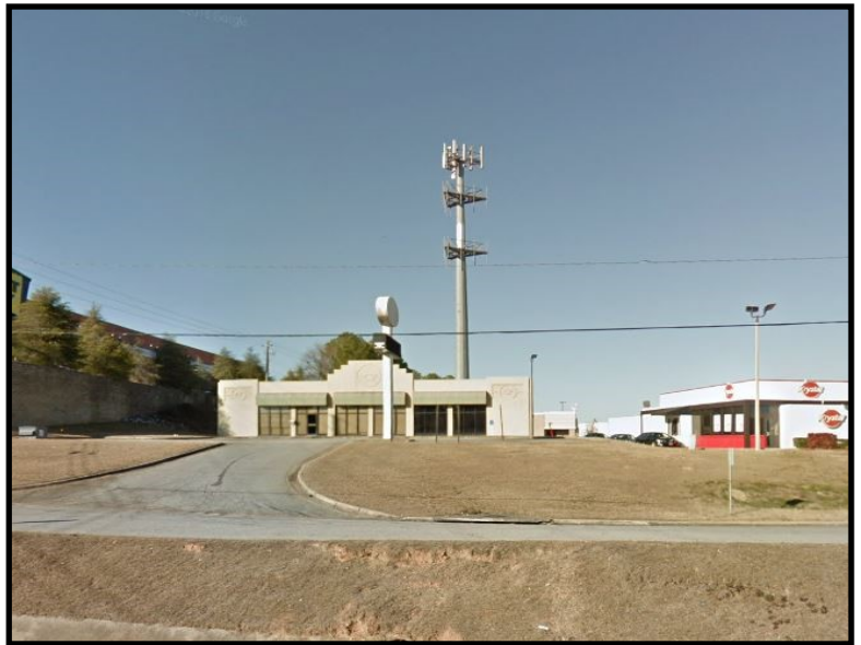
Cell Phone Tower along Manchester Expressway
