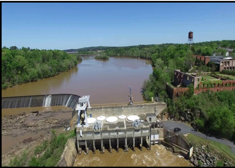
North Highlands Dam
