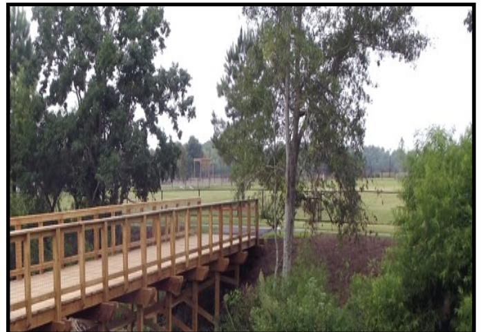
Oxbow Meadows Support Facility
