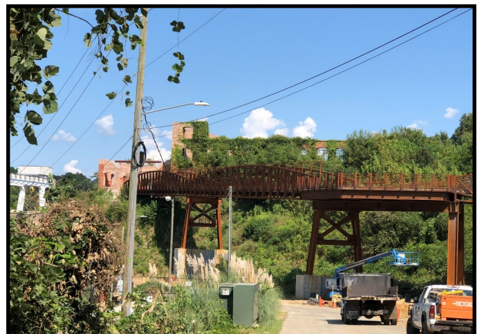
River Walk Bridge Expansion
