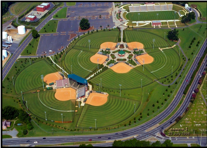
South Commons Baseball Complex
