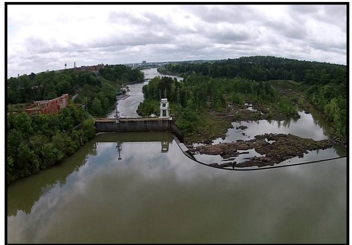
North Highlands Dam
