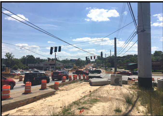
Talbotton Road Widening Project
