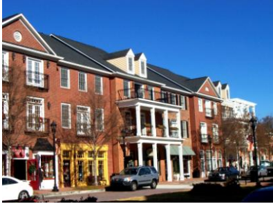
Smyrna Town Center in Smyrna, Georgia reflects the attributes of a village, reducing dependency on cars.
