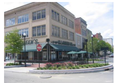
New housing within in-town neighborhoods will require higher densities to achieve financial feasibility.
