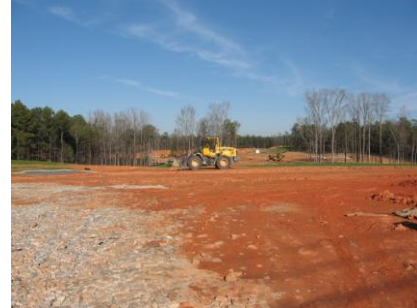
Construction site on Williams Road
