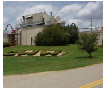
The City will need to dedicate funding for growth-related infrastructure to meet an increasing demand for services.
