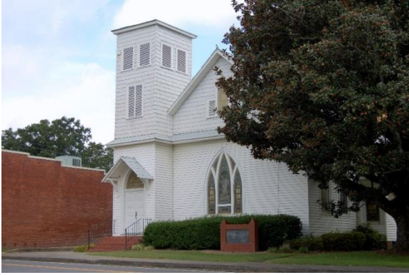
FIGURE 33. FIRST PRESBYTERIAN CHURCH OF COHUTTA, WOLFE STREET.
