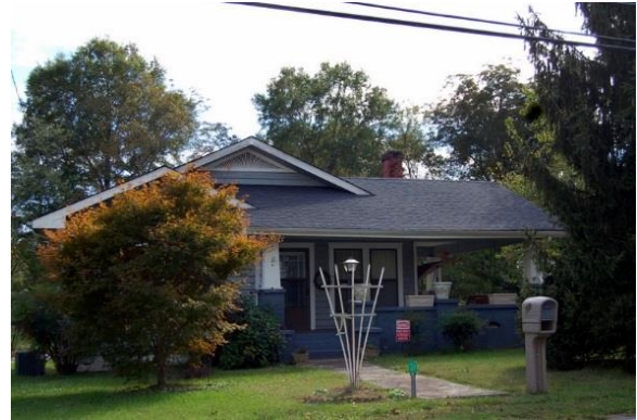
FIGURE 25. FRED RAINES HOUSE, WOLFE STREET
