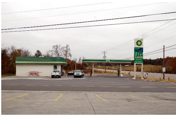
FIGURE 8. CLEVELAND HIGHWAY (RT. 71) AT THE INTERSECTION OF NORTH HILLS DRIVE
