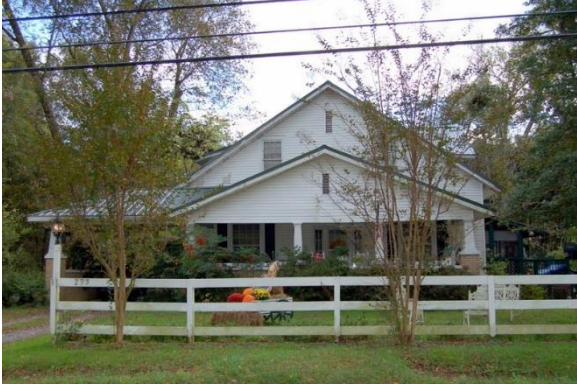
FIGURE 27. JOHN H. SHUGART HOUSE, WOLFE STREET
