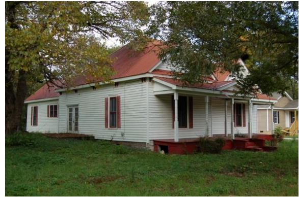
FIGURE 31. WATERHOUSE HOUSE, WOLFE STREET.
