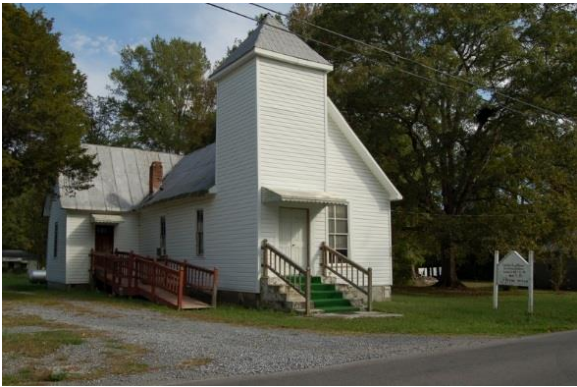
FIGURE 29. ST. ANDREWS CHAPEL METHODIST CHURCH, RED CLAY ROAD.
