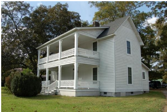
FIGURE 24. TOM BAGBY HOUSE, WOLFE STREET
