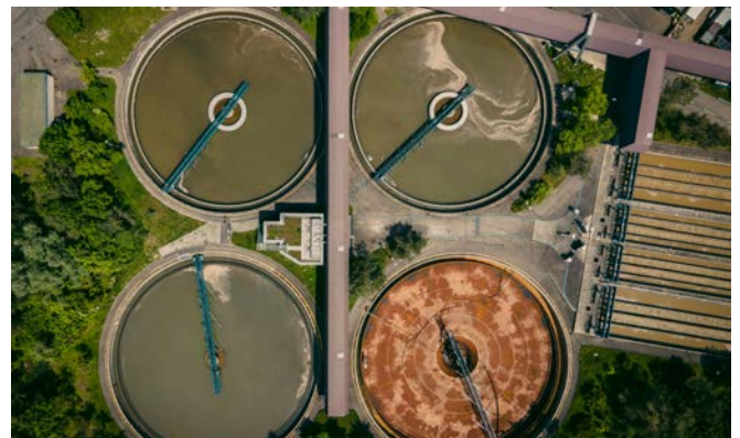
Image Caption: View of a sewerage treatment plant Source: Patrick Federi (2021)
