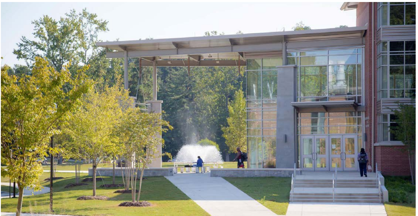
Image Caption: View of Lakeview Discovery and Science Center at Clayton State University Source: Clayton State University (2023)
