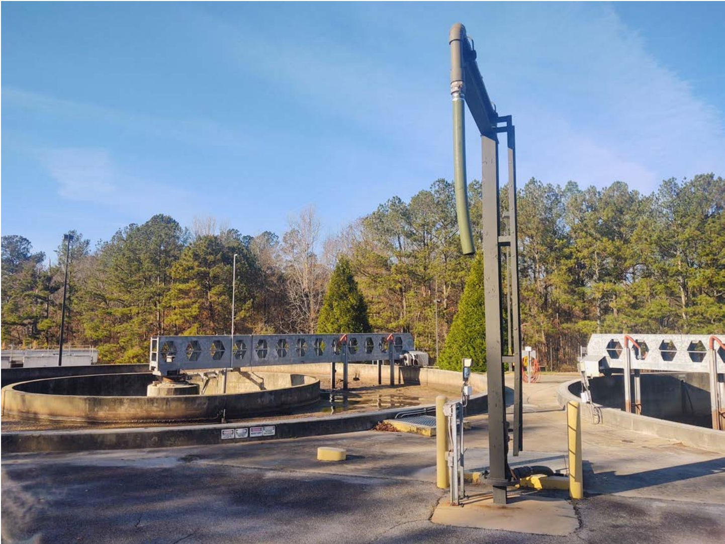
Image Caption: View of Clayton County Water Authority facilities (2024)
