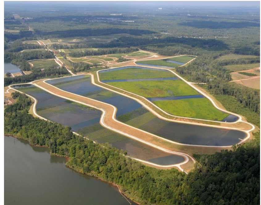
Figure 1 E.L. Huie Jr. Constructed Treatment Wetlands
