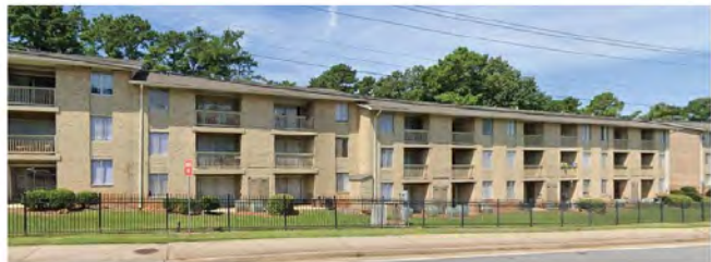
Aging multi-family buildings
