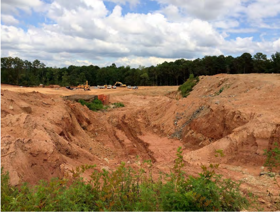
Site work in progress.
