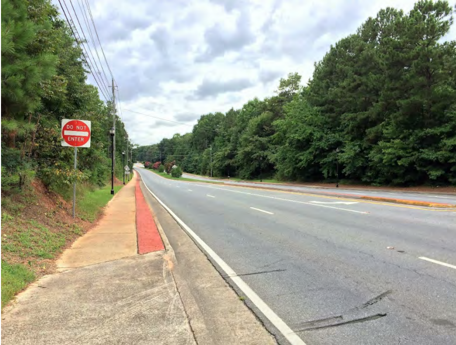
Wade Green Road streetscape improvements. The tract is located on the left. A curb cut for the tract can be seen in the lower left corner.
