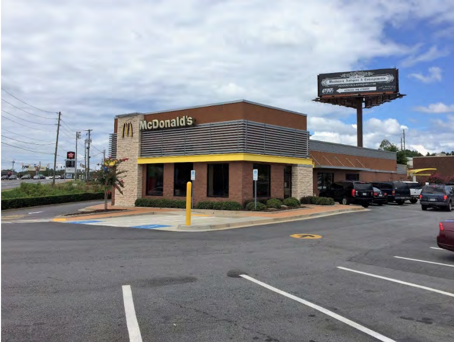
Façade and site improvements.
