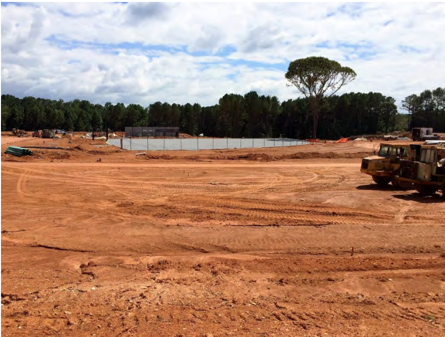
Site work in progress.
