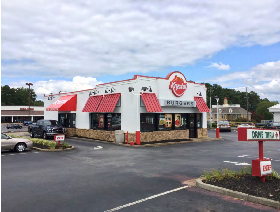
Façade and site improvements.
