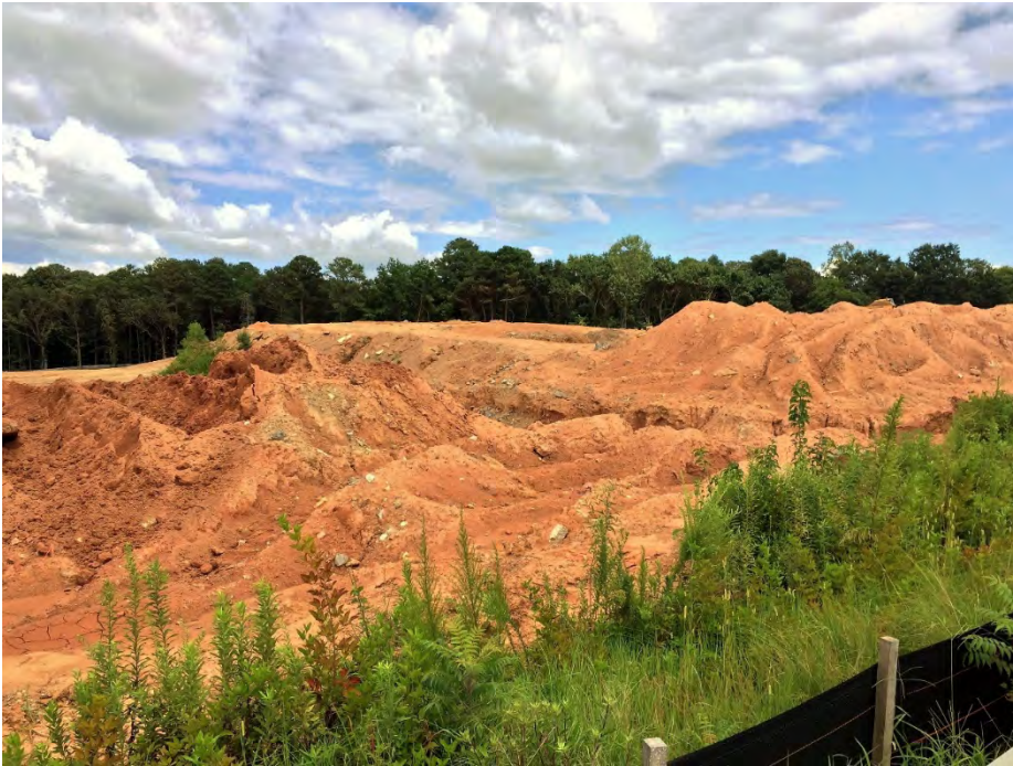
Site work in progress.
