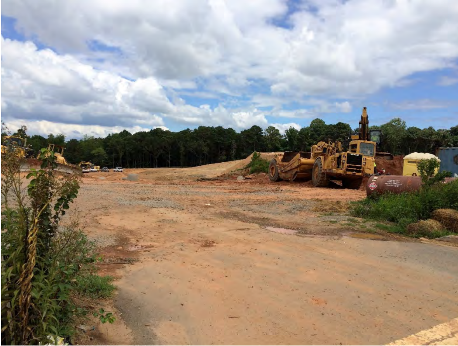
Site work in progress.
