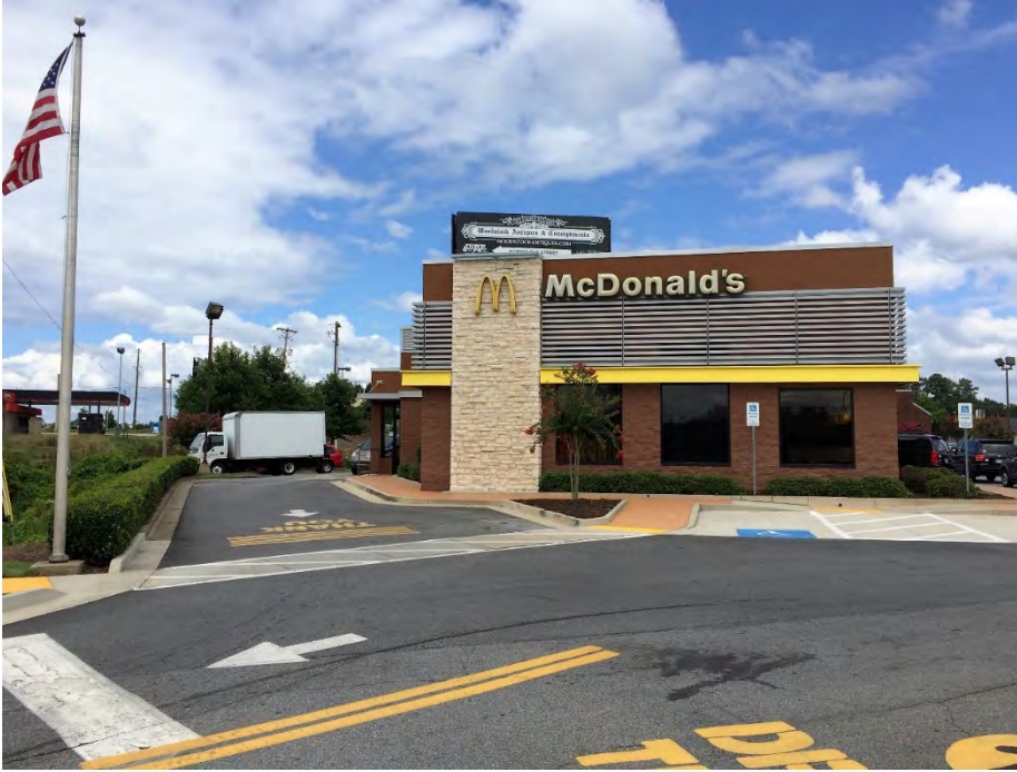
Façade and site improvements.
