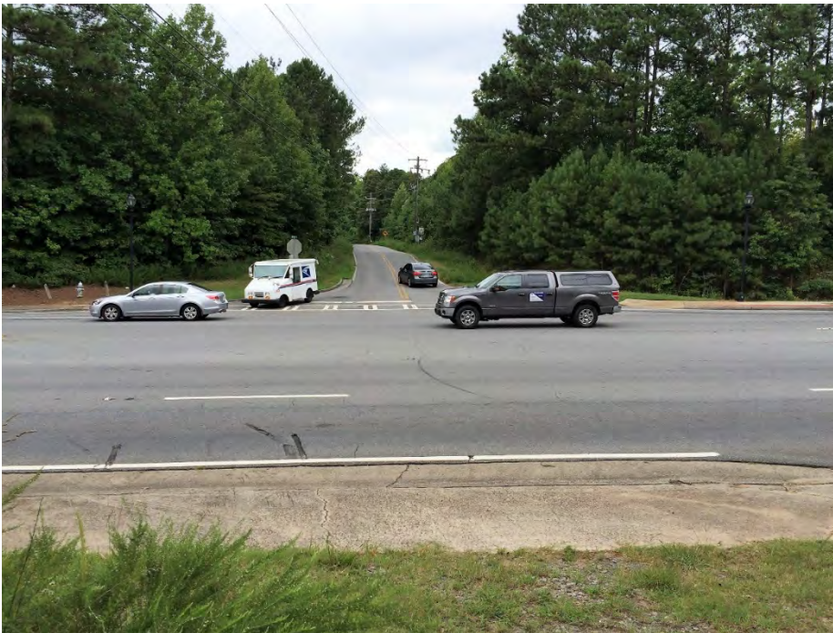
A median break on Wade Green Road at Hopgood Road will improve access to the site. A curb cut for the tract is visible at the bottom.
