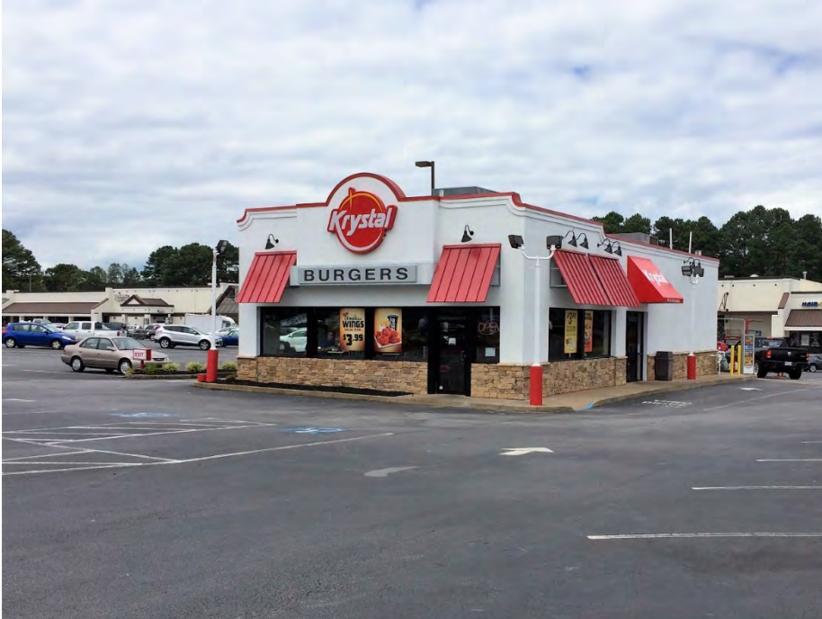
Façade and site improvements.
