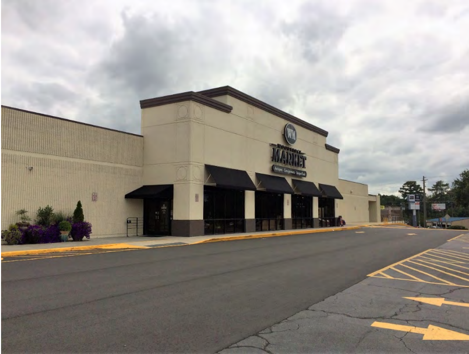
Woodstock Market – façade improvements.
