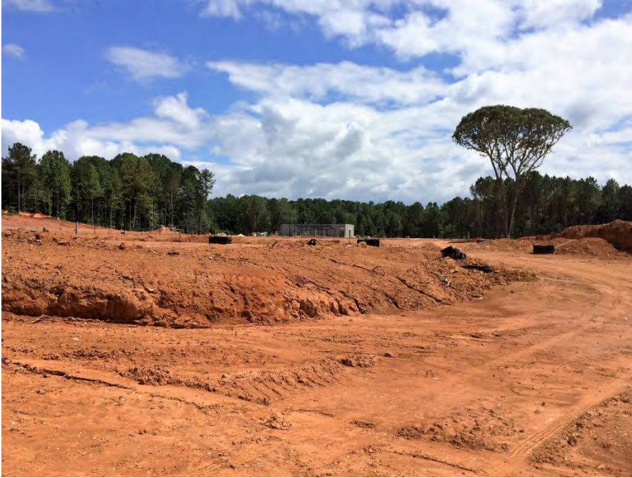
Site work in progress.
