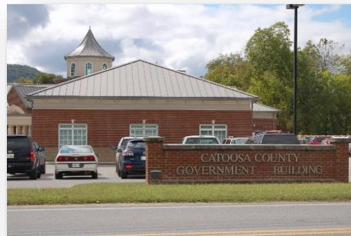
Figure 6. Catoosa County Government Building, Ringgold.
