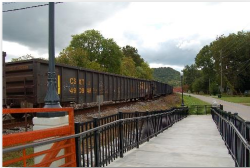
Figure 14. Train at Ringgold Depot.
