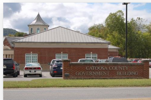
Figure 6. Catoosa County Government Building, Ringgold.
