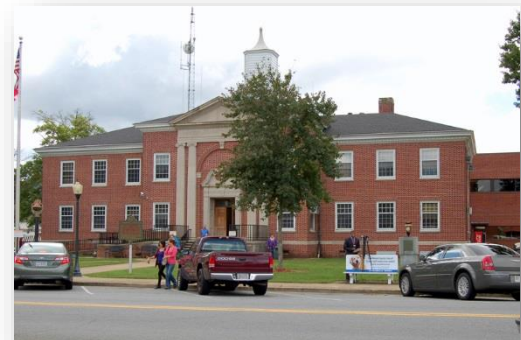
Figure 18. Catoosa County Courthouse, Ringgold.
