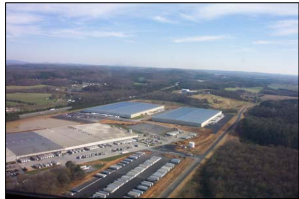
The Mohawk Plant off of Union Grove Road, Calhoun
