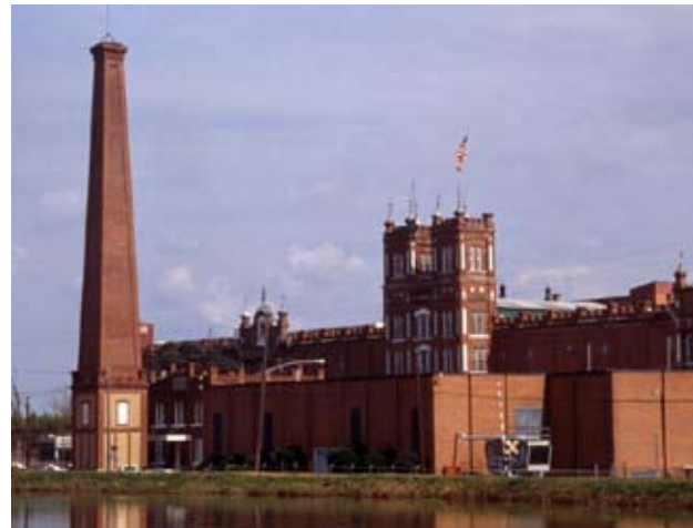
Top: Enterprise Mill, constructed in 1877–88, and part of the Augusta Canal NHL and heritage area, was rehabilitated using federal historic preservation tax credits. It now hosts businesses, apartments, and a state of the art museum and interpretive center that attract thousands of visitors a year. Bottom: MLK Birth Home, listed in the National Register of Historic Places and a National Historic Landmark, is visited by both national and international travelers because of its association with Martin Luther King, Jr., the pivotal figure of the 1960s civil rights movement.
