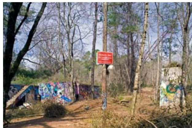
Decatur Waterworks, located in DeKalb County and listed in the National Register in 2006, was completed in 1907, and became a park in 1942. It is significant in landscape architecture as a planned park.
