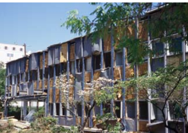
The Alcoa building in Atlanta, an International style building composed of an extensive aluminum panel system, was built in 1955 to showcase interior and exterior applications of aluminum. It was demolished in 2004.
