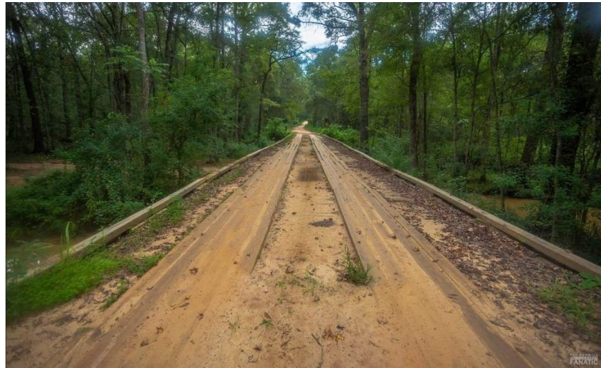
Figure 2. Mule Creek Bridge Quitman, GA, Source: The GA Photography Fanatic; http://forgottengeorgia2.blogspot.com/2018/08/mule-creek-bridge.html
