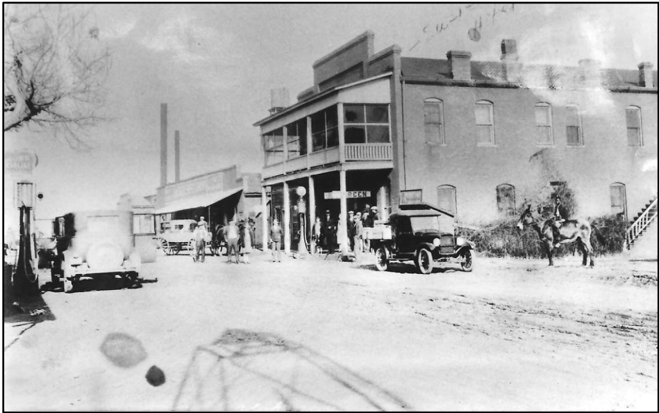
Figure 4 Streetscape photograph of downtown Bostwick, 1927. Collection of Morgan County Archives. This photograph reveals many elements of historic downtown Bostwick which are extant, including the Susie Agnes Hotel and the General Store. In the distance, the smoke stacks of the manufacturing plant (now demolished) are visible and the shadow of what may be a fire alert bell appears in the foreground.
